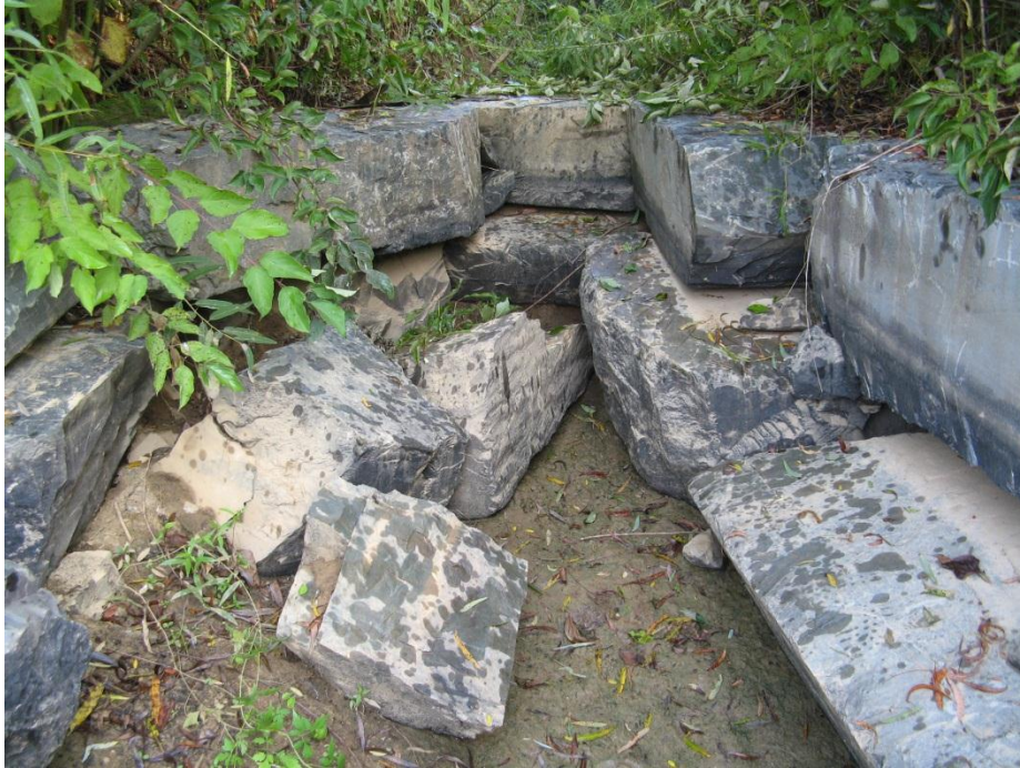
Problem Area 7 Photo
