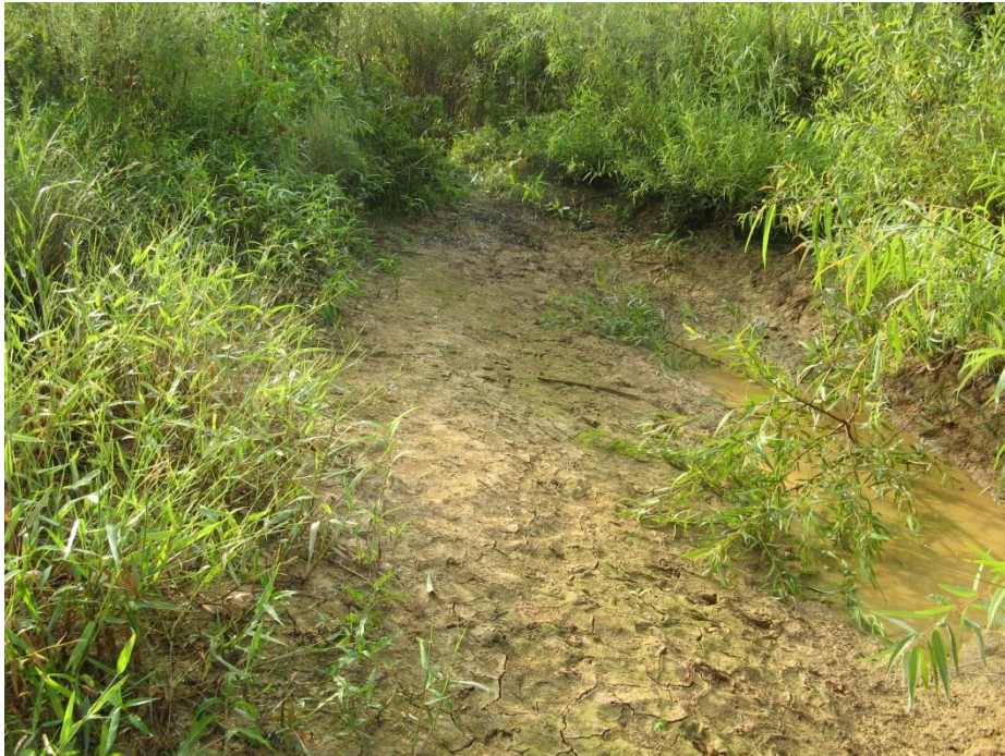
Problem Area 4 Photo
