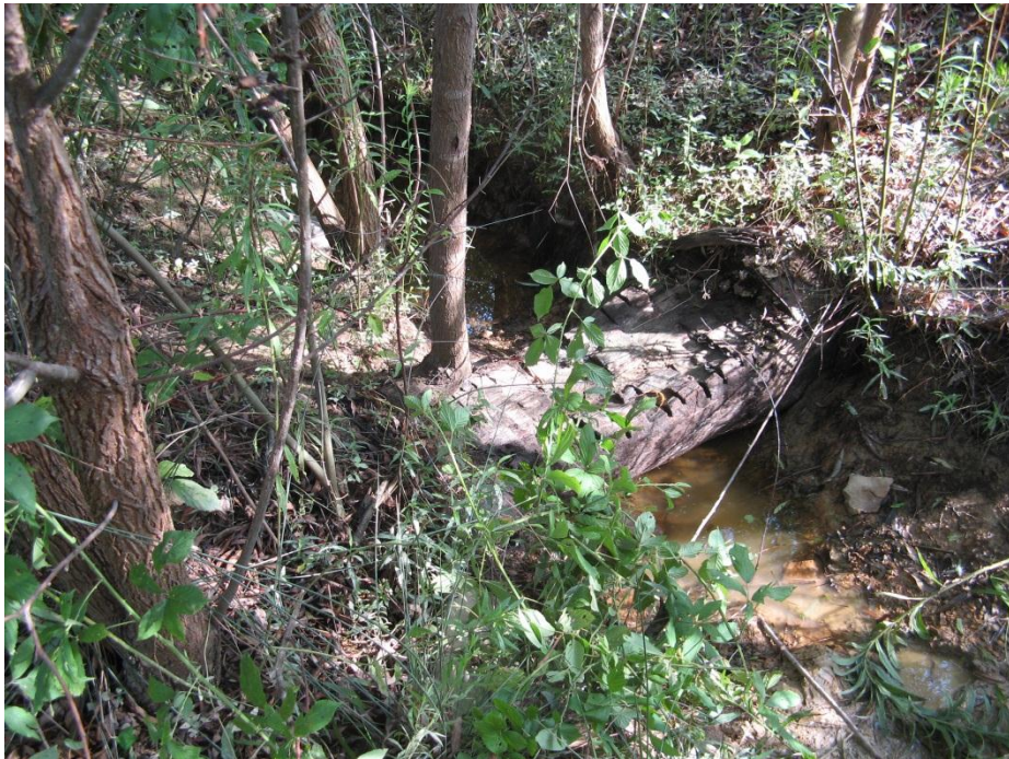
Problem Area 6 Photo
