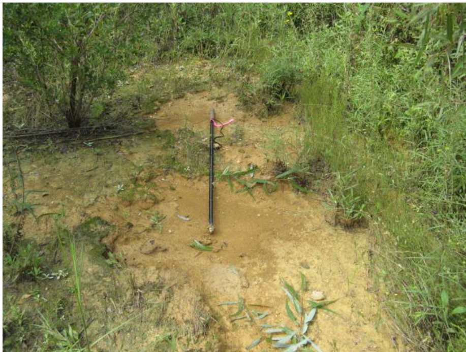
MY2_PA3 - Diversion channel 45 feet of left bank from channel blockage
