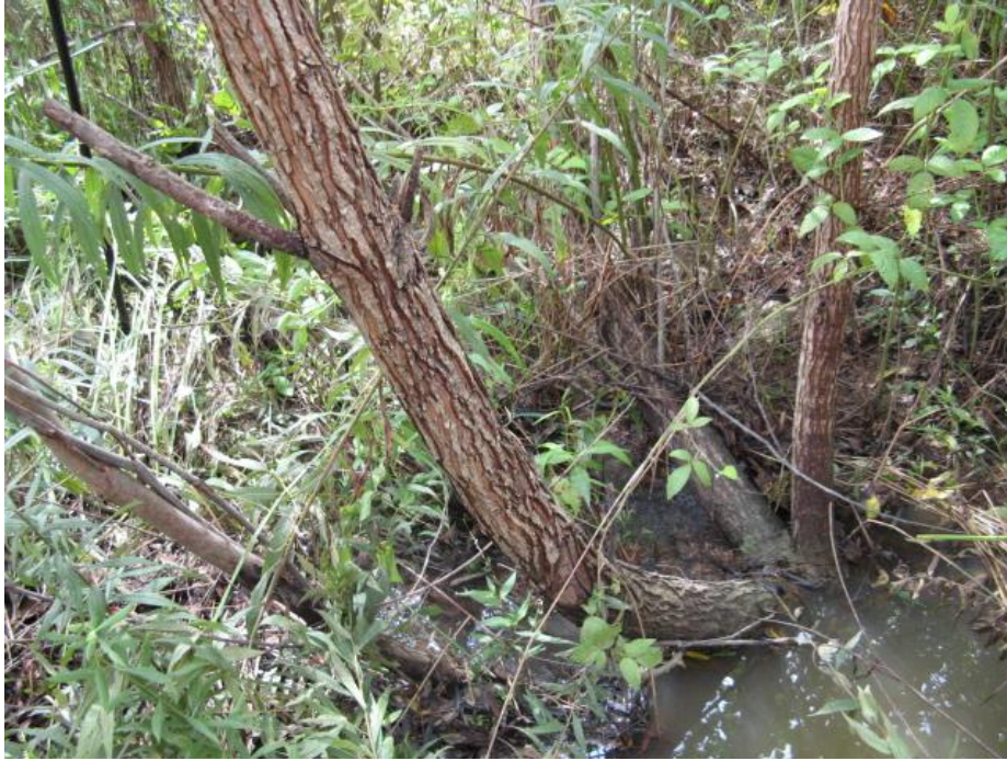
MY4-PA11 Channel obstruction
