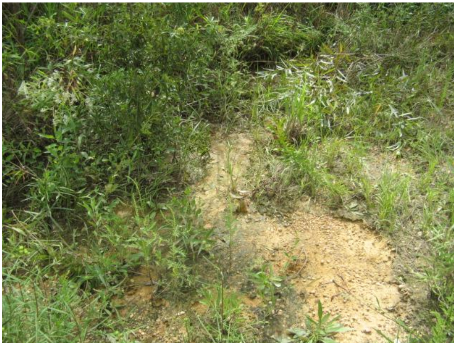
MY5-PA2 - Diversion channel cutting 40 feet of right bank from channel blockage
