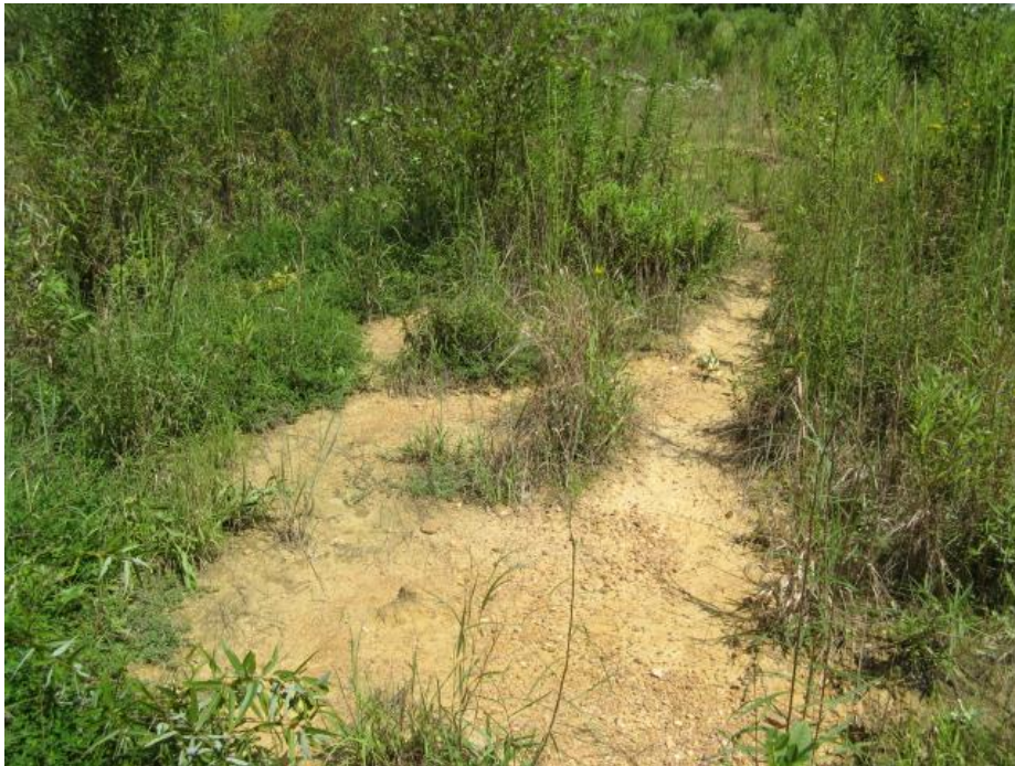
MY4-PA8 Diversion channels cutting 140 feet of both banks, no woody vegetation
