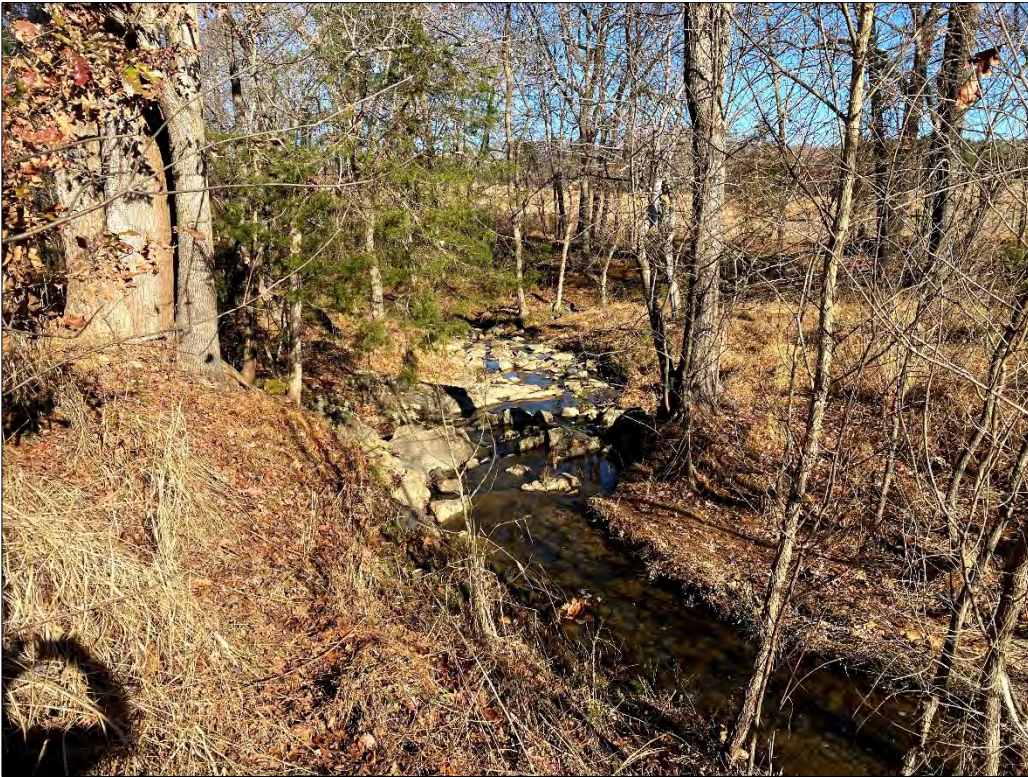
Mainstem Near XC 20, Transition from Restoration to Enhancement 2
