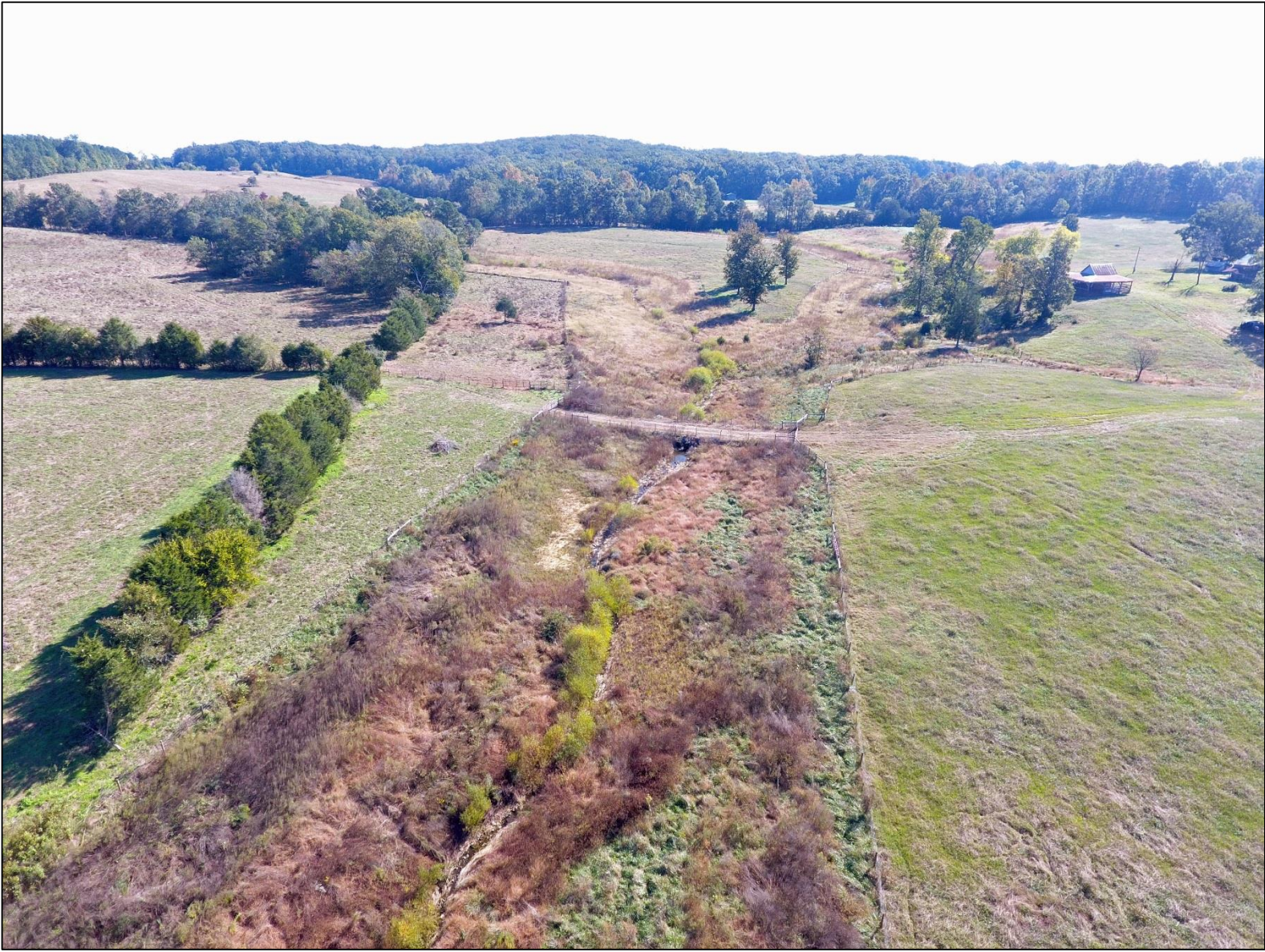
Photo 6: middle crossing looking upstream at the Main Stem and UT-3 on the left
