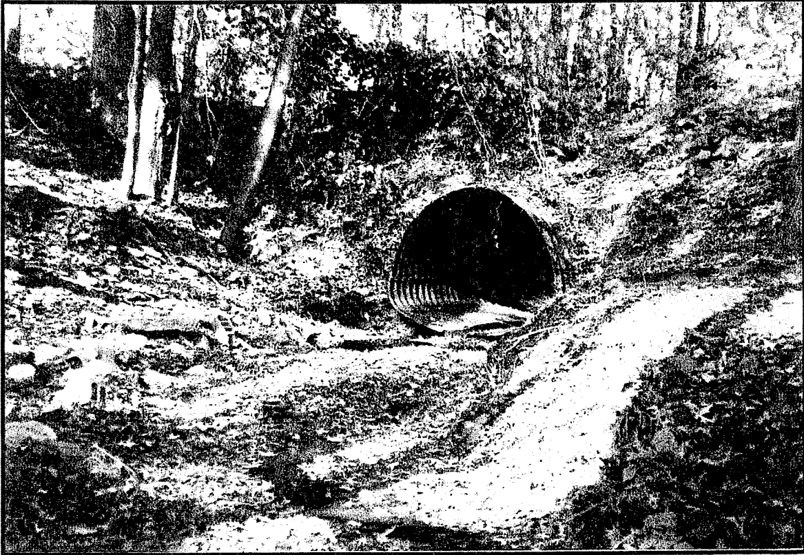
1. Culvert under Lakeside Drive. (Upstream View)
