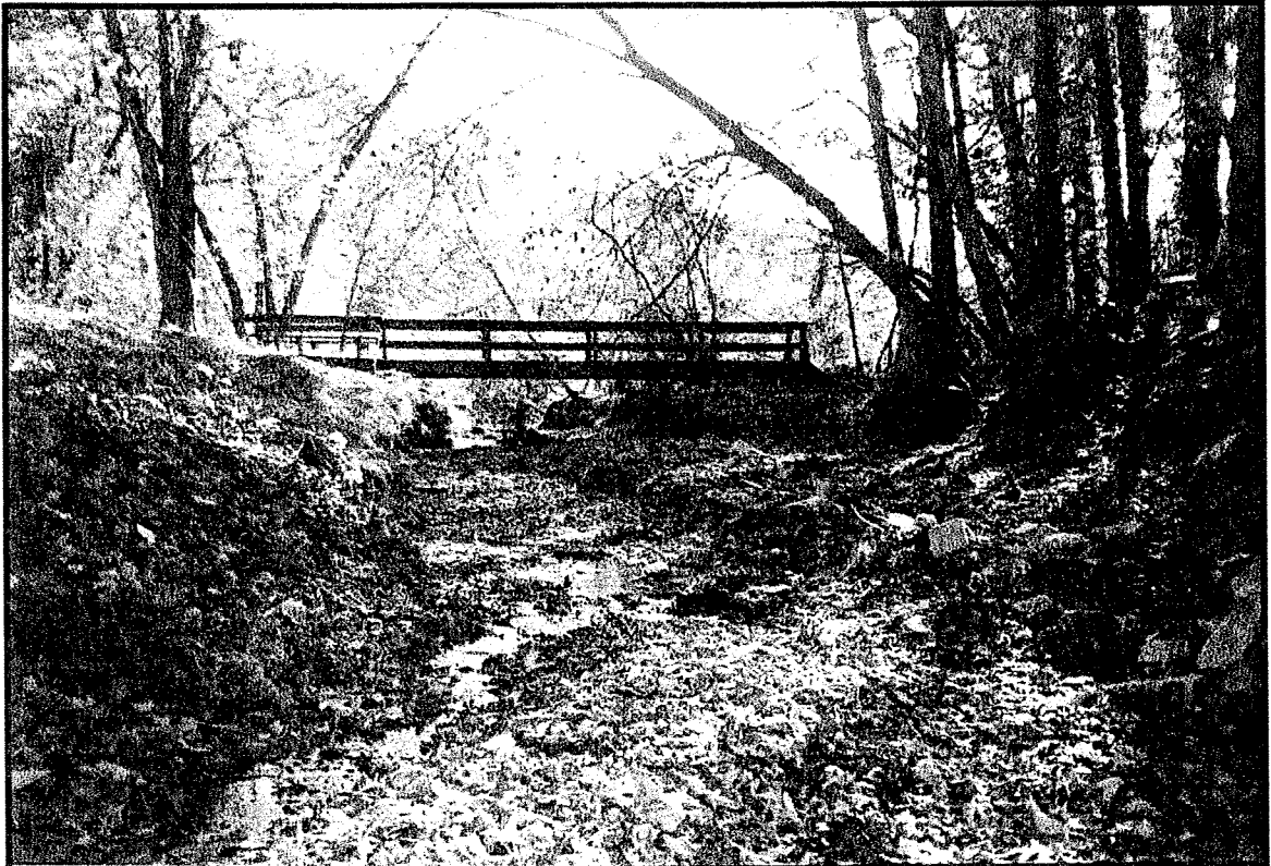
2. Wooden foot bridge in picnic area. (Downstream View)
