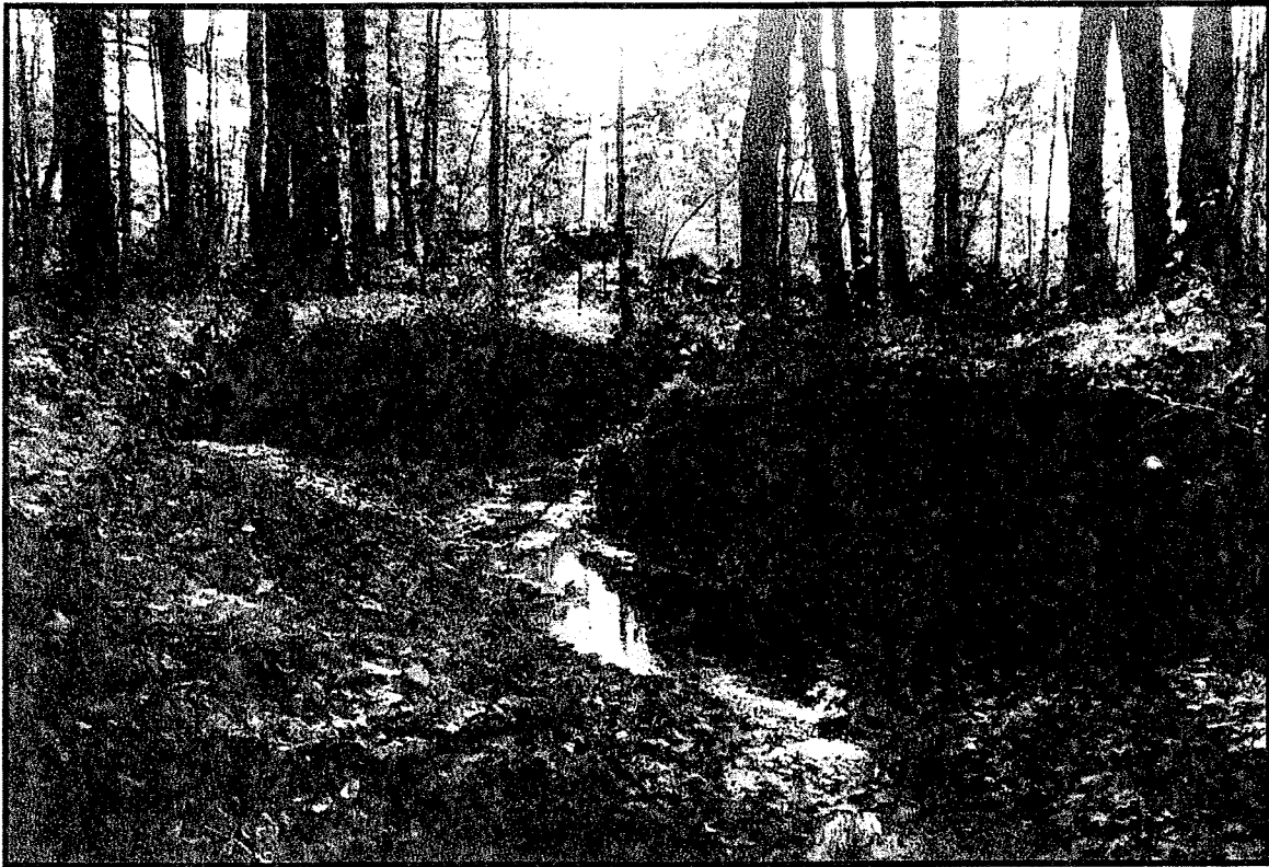
9. Bank erosion downstream of dam.
