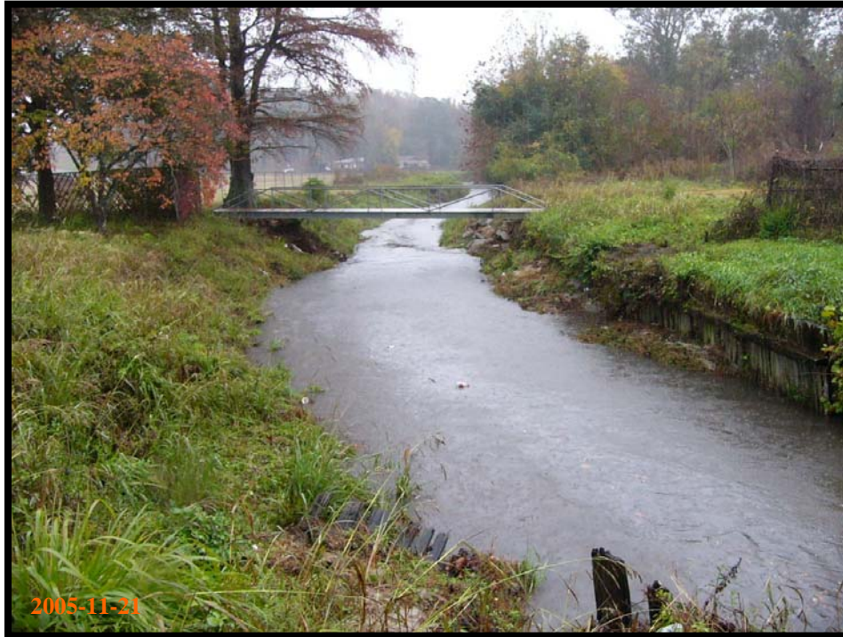
Existing Pedestrian Bridge near Washington Street
