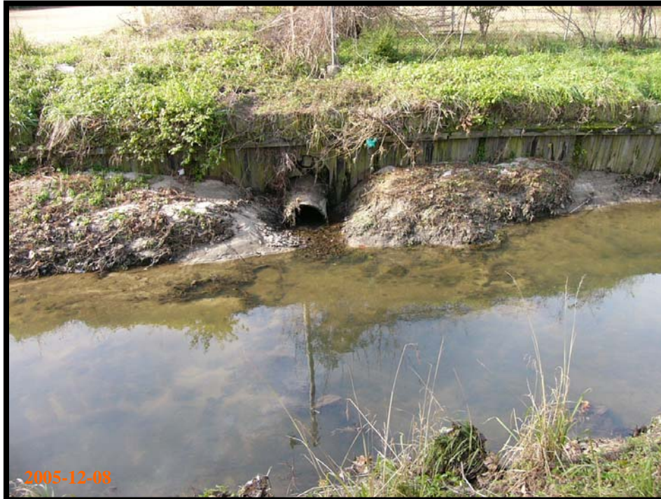
Existing Storm System Outfall
