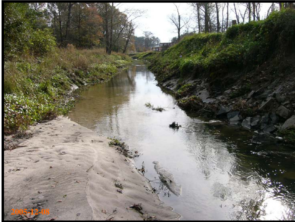
Adkin Branch Looking Downstream near Charter School
