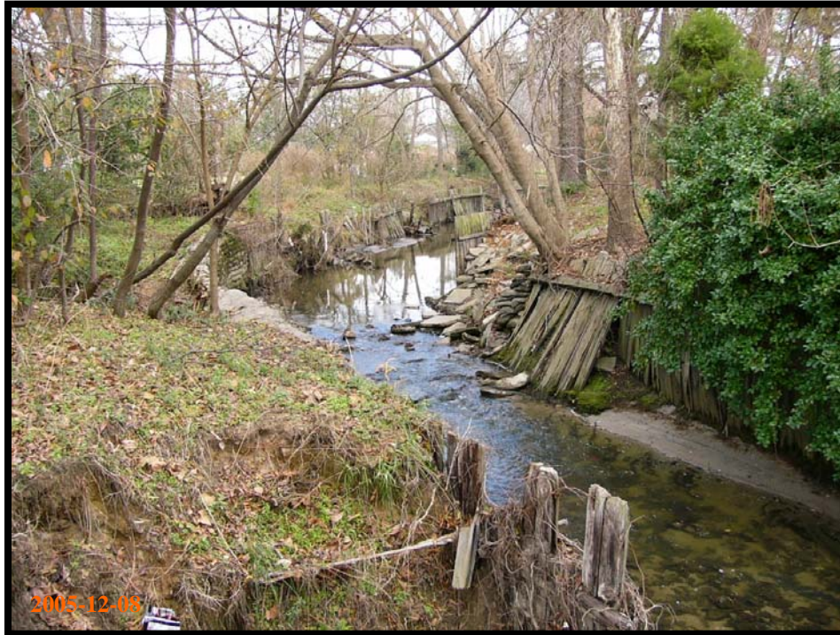
Adkin Branch Looking Upstream near Gordon Street
