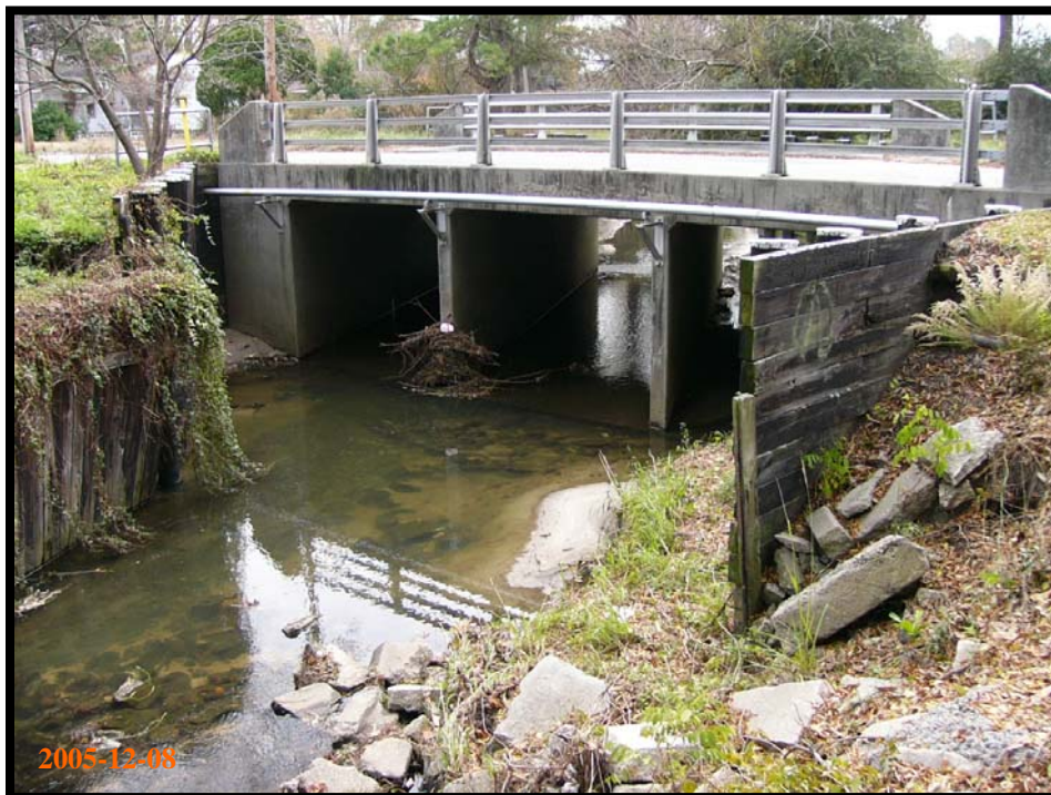
Existing Culvert Crossing with Timber Retaining Walls
