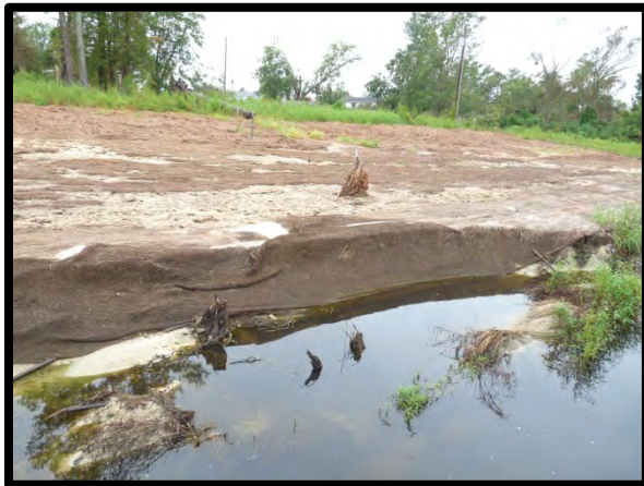
3.25 Severe erosion/bare benches near 83+00
