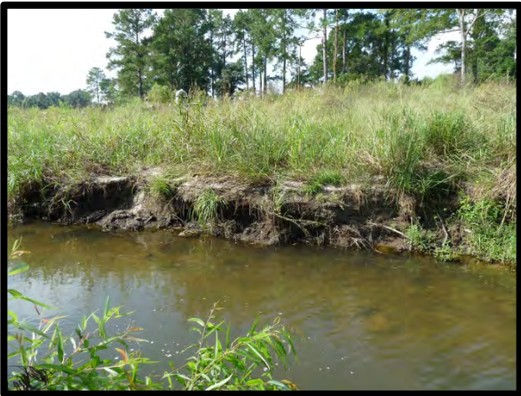
3.24 Severe erosion near 86+70
