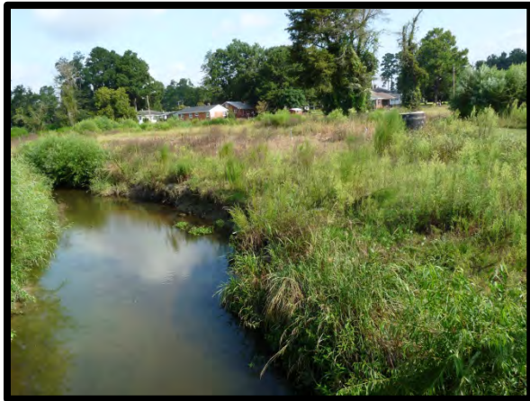
3.23 Severe erosion upstream of pedestrian bridge (83+50)
