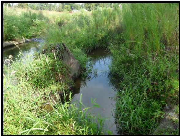
3.30 Severe erosion around vane arm 2012 (87+50)
