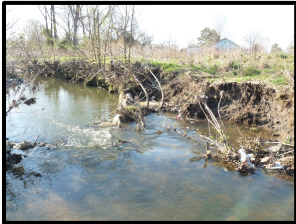
3.23 Scouring on log vane XS 6
