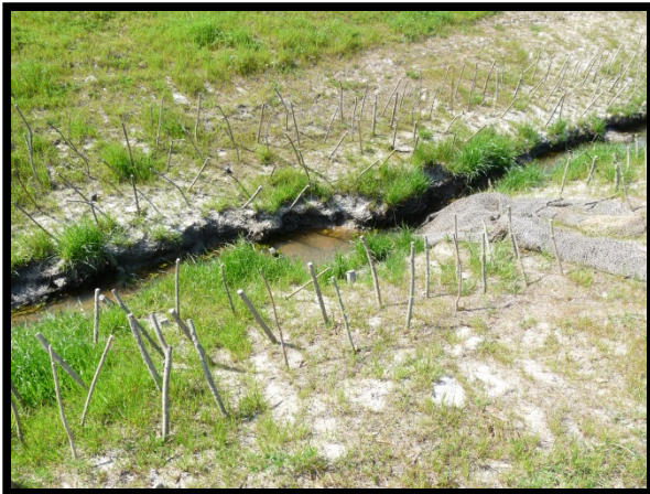
3.27 Live Stakes on BMP Channel
