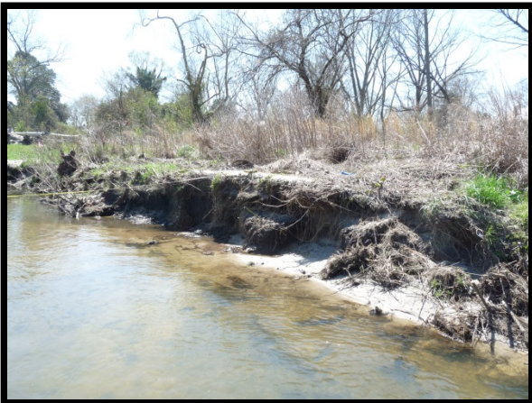
3.28 Scouring at XS 9
