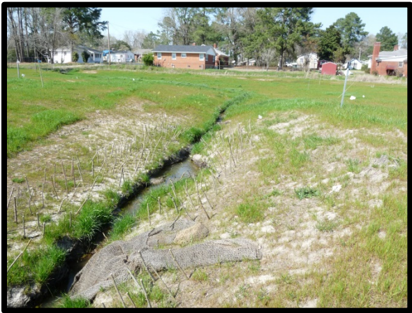
3.29 Live Stakes on BMP Channel
