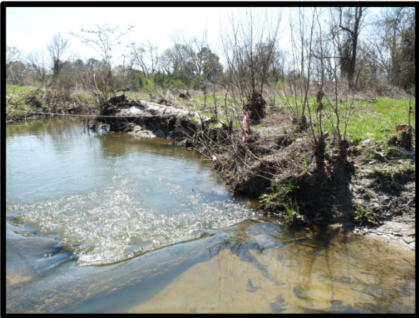
3.24 Scouring on log vane XS 8
