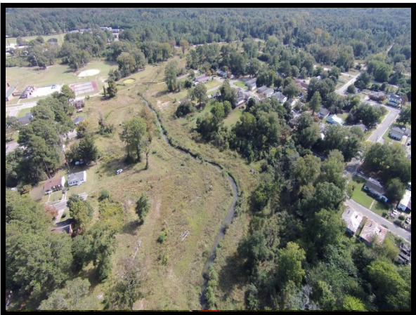
3.32 Looking Downstream at Holloway Park
