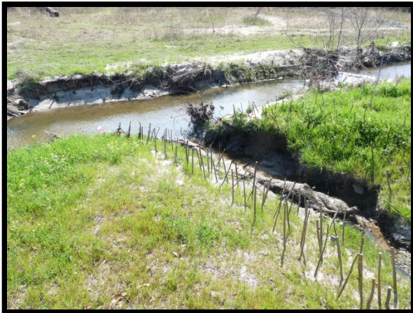
3.28 Live Stakes on BMP Channel
