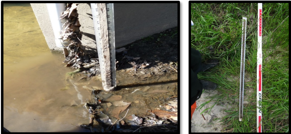
Figures 8.11 - 6.12 2014 & 2015 Crest Gauge Photos
