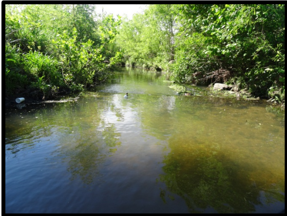
3.29 Stress structure near 62+10
