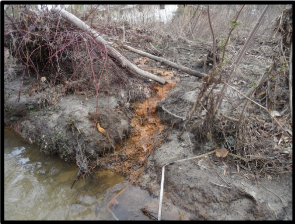
3.24 Overflow channel from drainage ditch off Sycamore Street near 47+30
