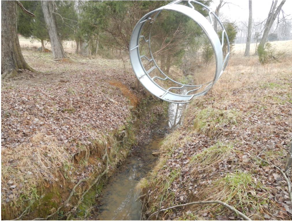
Photo 7. UT1A Reach 1 - Restoration
