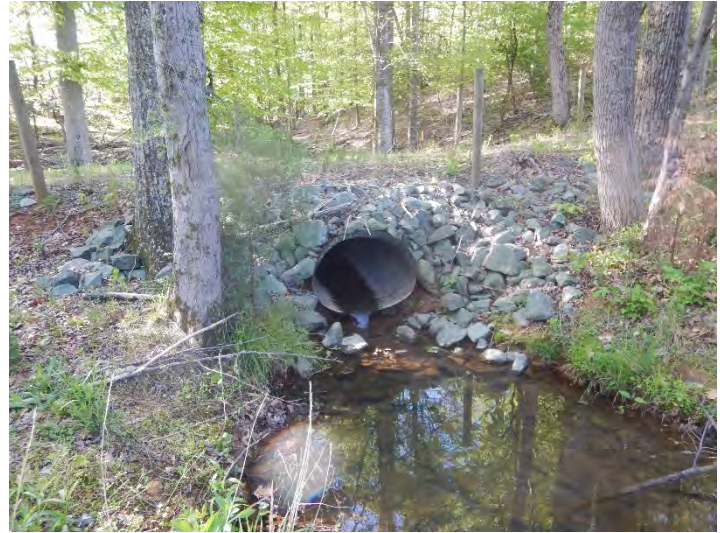
UT1A Perched Culvert – (04/17/2020)
