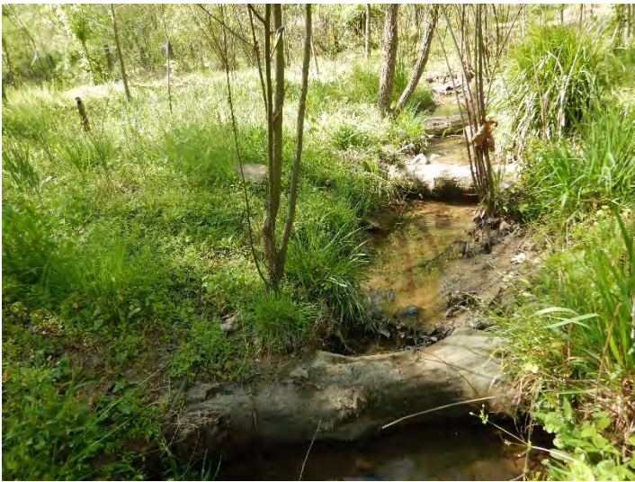
UT2 Piping Log Sills – (04/17/2020)
