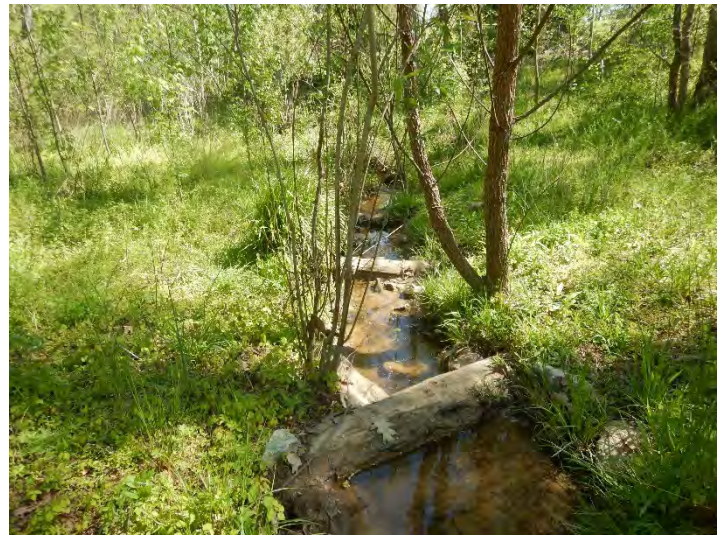
UT2 Piping Log Sills – (04/17/2020)
