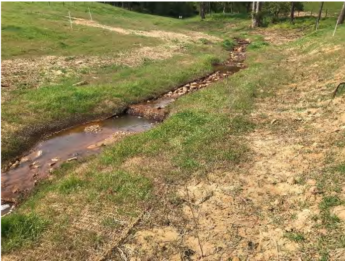
PP5 – view upstream- UT1 Reach 1B (04/22/2020)
