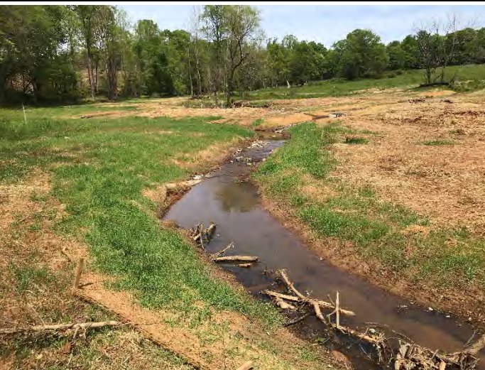
PP15 – view upstream— UT1 Reach 4B (04/22/2020)
