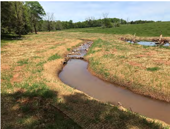
PP17 – view upstream— UT1 Reach 4B (04/22/2020)
