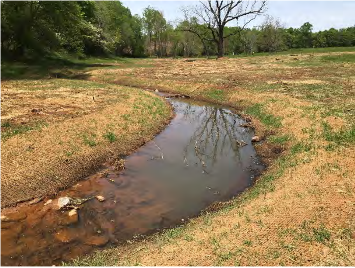
PP16 – view upstream— UT1 Reach 4B (04/22/2020)
