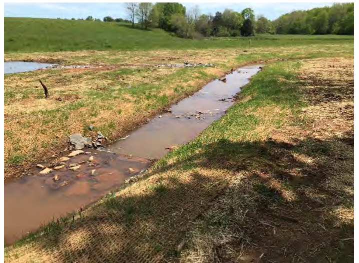
PP17 – view downstream— UT1 Reach 4B (04/22/2020)
