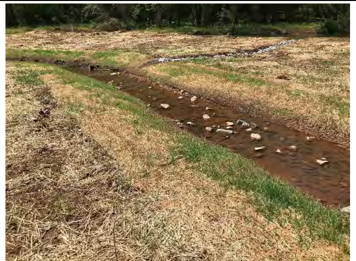
PP18 – view downstream— UT1 Reach 4B (04/22/2020)
