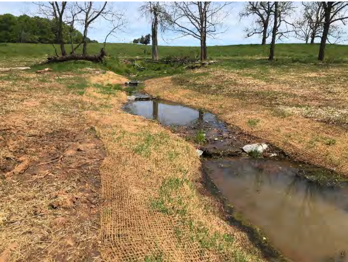
PP20 – view upstream— UT1A (04/22/2020)
