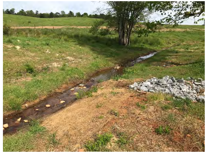
PP6 – view downstream—UT1 Reach 1B (04/22/2020)
