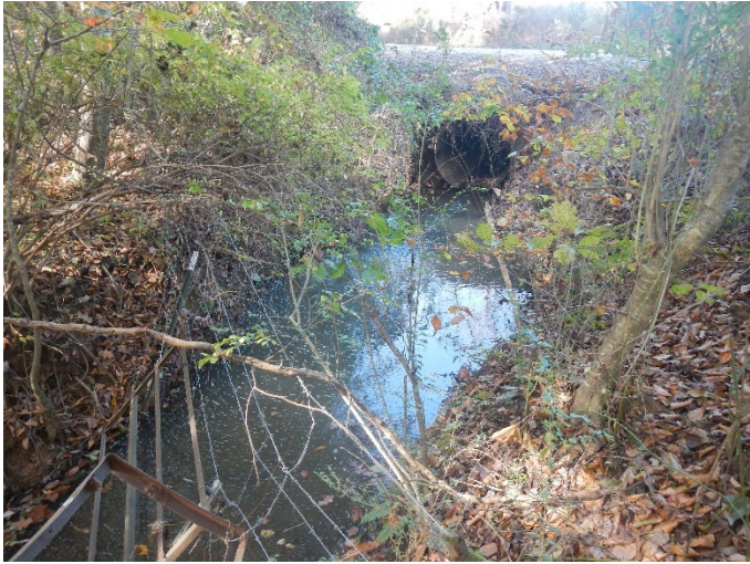
PP9B – view upstream—UT1 Reach 3 (11/05/2020)
