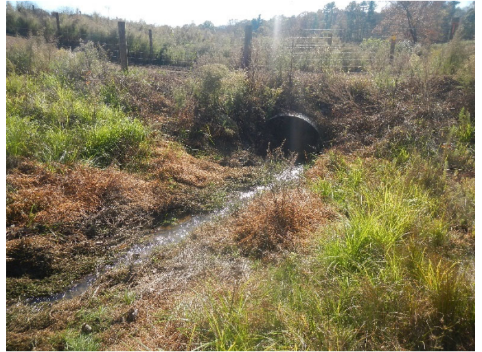
PP6A – view downstream—UT1 Reach 1B (11/05/2020)
