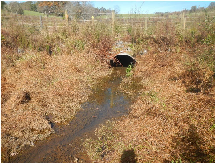
PP6B- view upstream—UT1 Reach 2 (11/05/2020)
