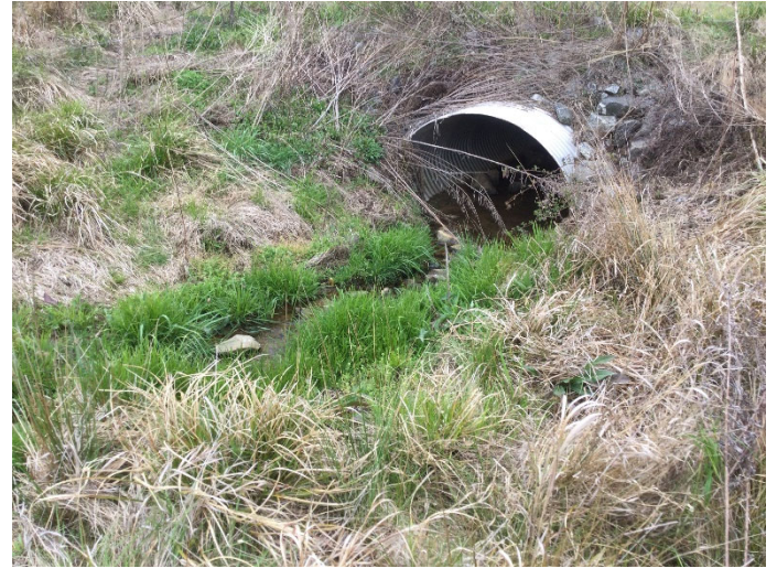
PP6A – view downstream—UT1 Reach 1B (04/05/2022)
