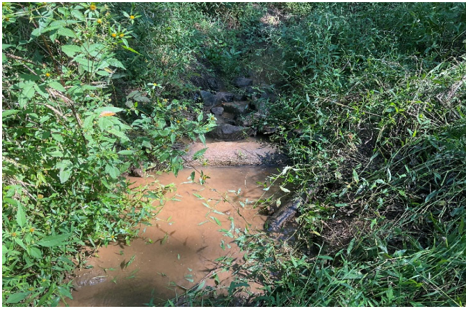
UT1 R1A Structure Piping (STA 104+00) – view upstream (09/20/2022)
