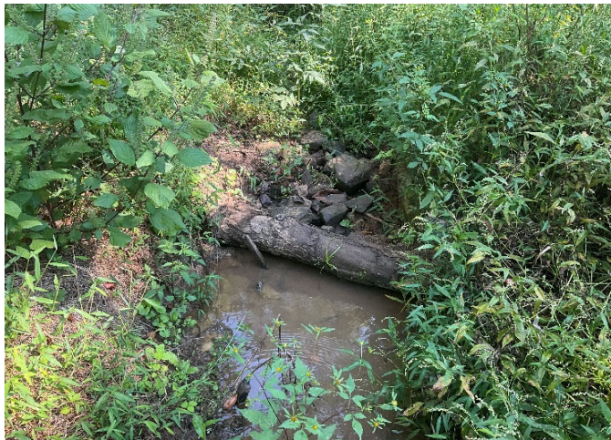
UT1 R1A Structure Piping (STA 104+05) – view upstream (09/20/2022)
