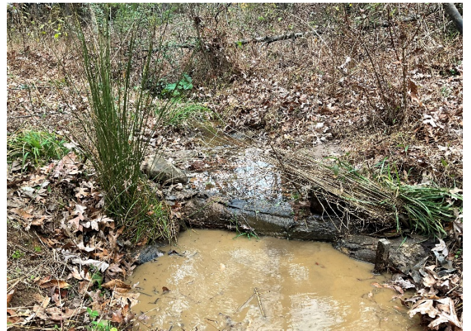
UT1 R1A Structure Repaired (STA 104+05) – view upstream (11/10/2022)
