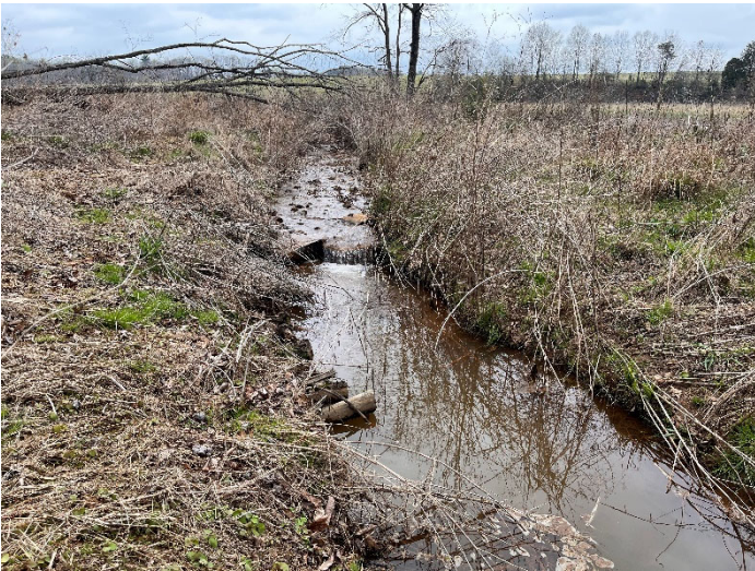
PP19 – view upstream— UT1 Reach 4B (04/05/2022)
