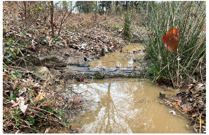
UT1 R1A Structure Repaired (STA 104+00) – view upstream (11/10/2022)
