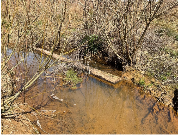
PP21 – view upstream— UT1 Reach 4B (03/09/2023)
