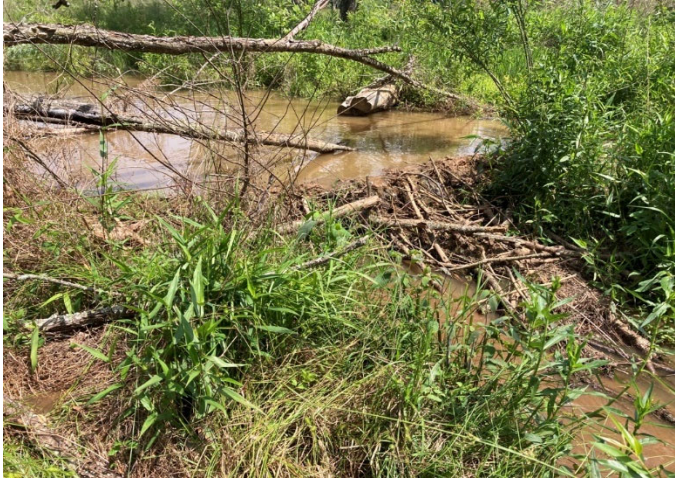
Beaver Dam – view upstream – UT1 R4B at STA 165+58 (05/10/2023)
