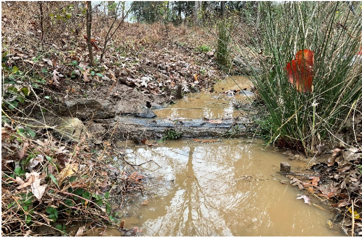
UT1 R1A Structure Repaired (STA 104+00) – view upstream (11/10/2022)
