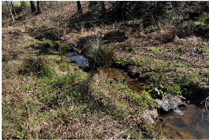
UT1 R1A Structure Repaired (STA 104+00 – 104+05) – view upstream (03/09/2023)
