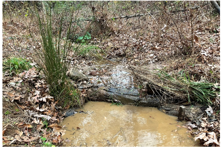
UT1 R1A Structure Repaired (STA 104+05) – view upstream (11/10/2022)
