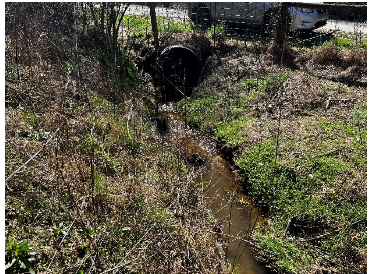
PP9A – view downstream—UT1 Reach 2 (03/09/2023)
