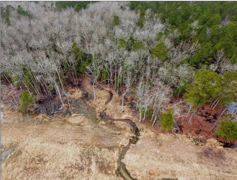
Eastern Easement, UT-3 origin point, 12/22/2019
