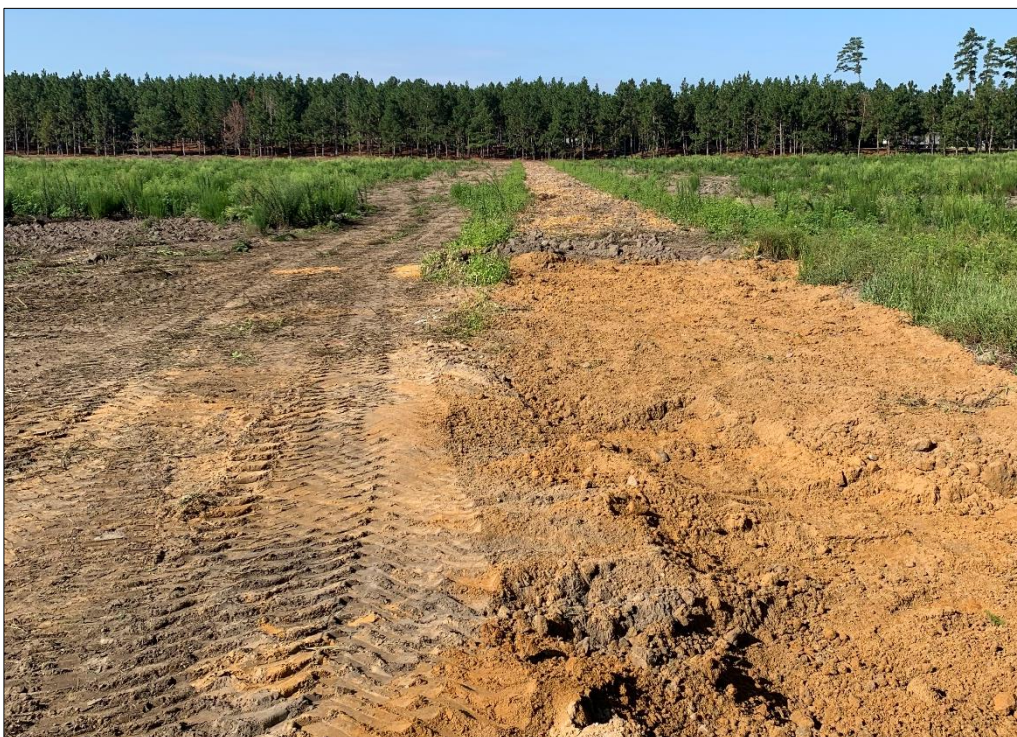
Filled ditch looking south near Project's outfall - 08/8/2019
