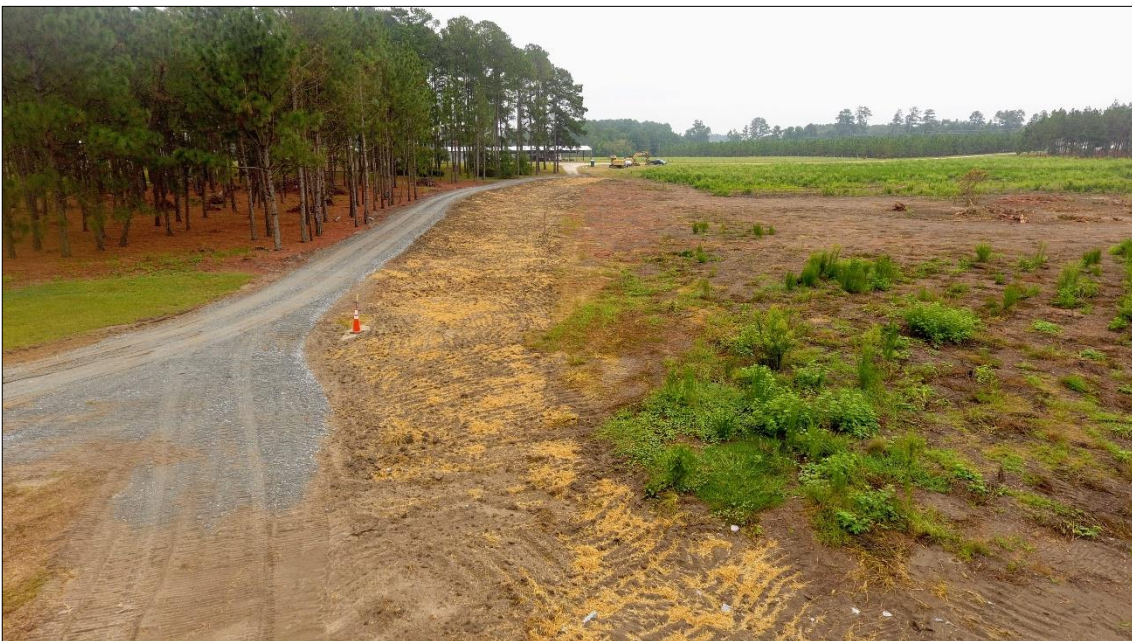
New road, old road, looking east from Project outfall - 08/15/2019
