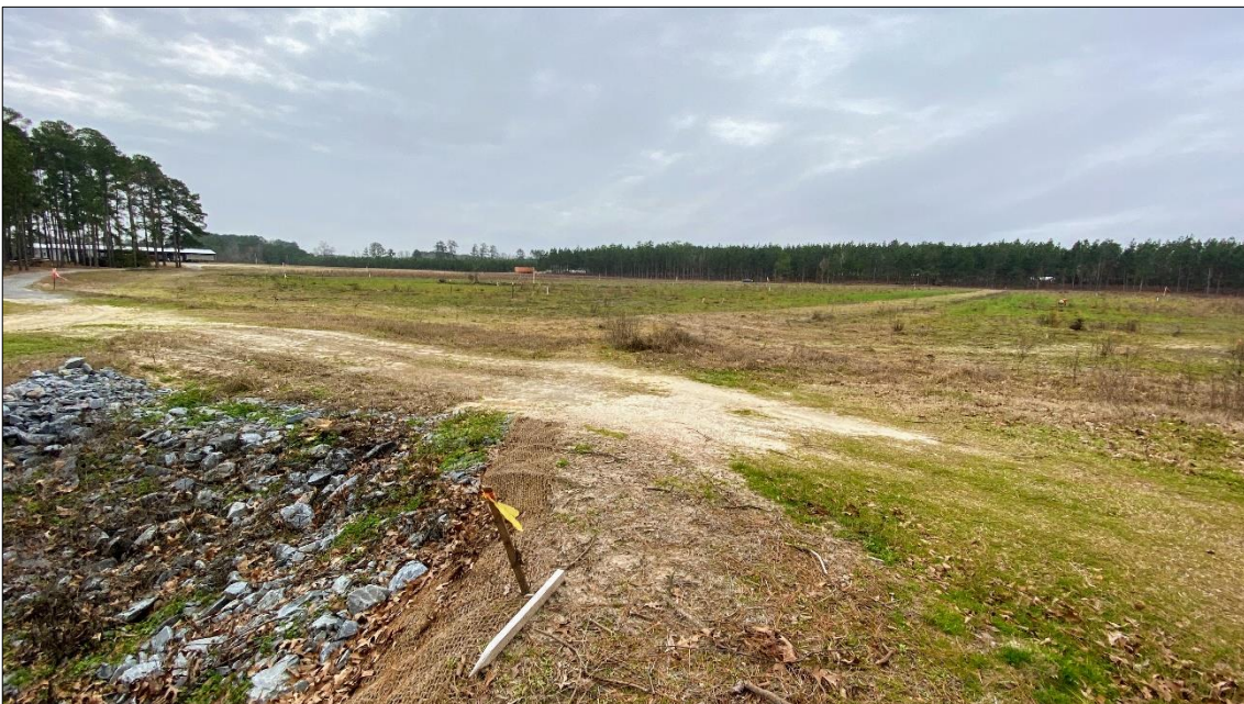
Project outfall looking southeast across the Site - 01/24/2020
