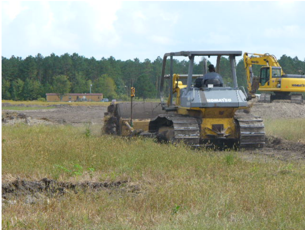
Photo 3. Initial cutting and stockpiling of topsoil for redistribution after final grading.
