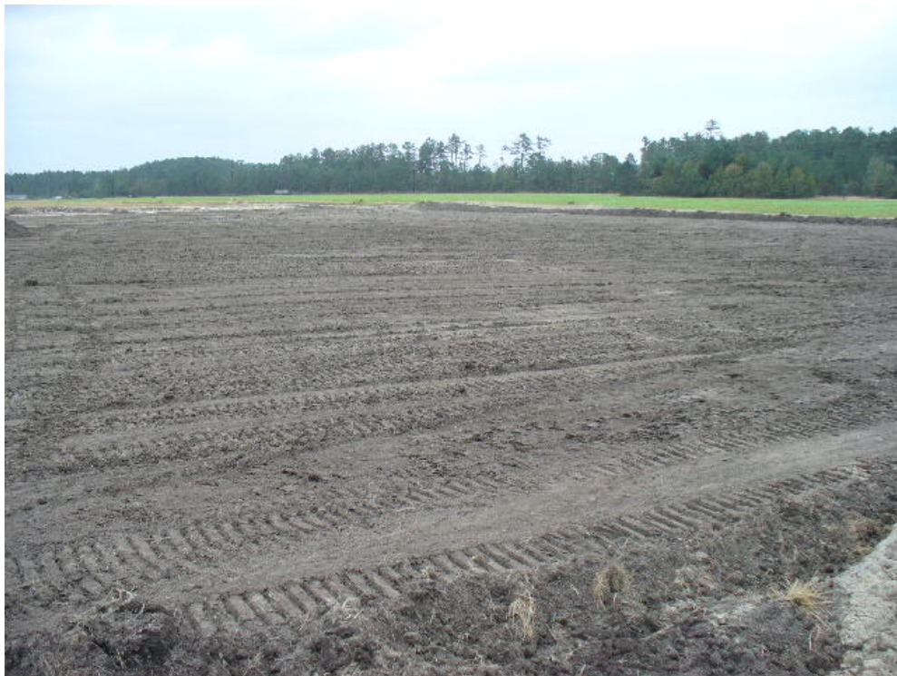
Photo 6. Restored swamp run after final grading.
