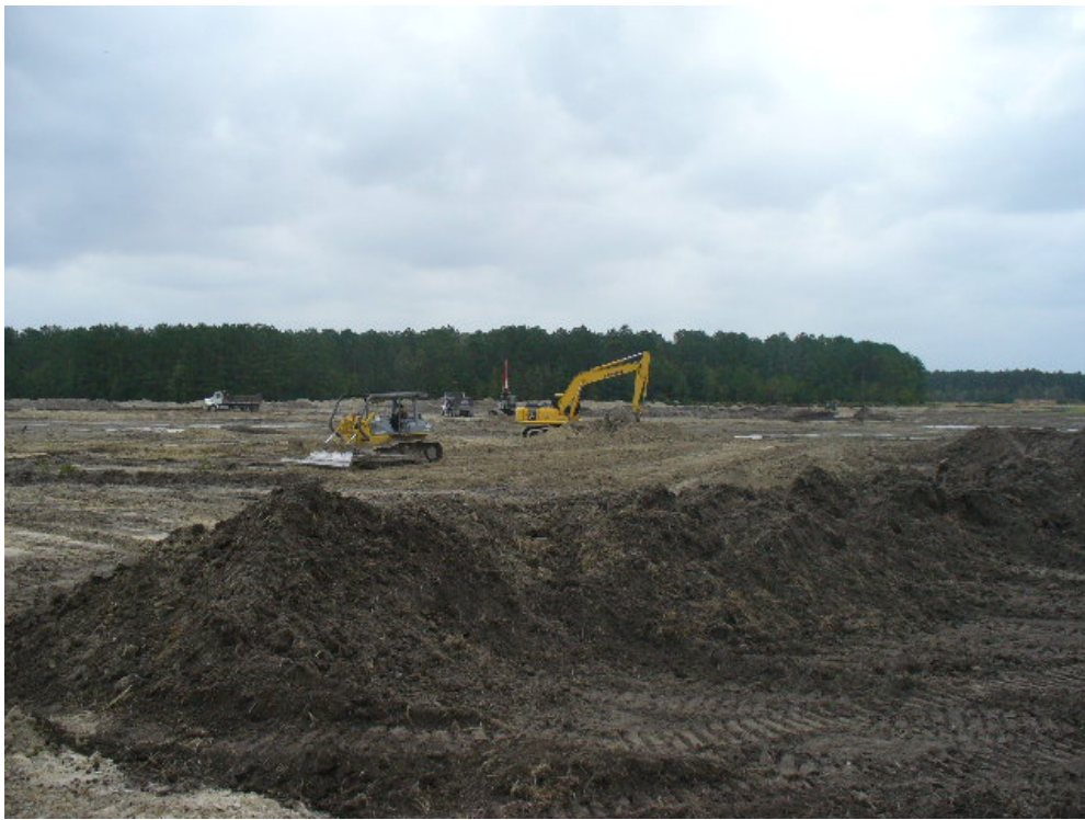
Photo 4. Cutting, filling and grading of restore swamp run.
