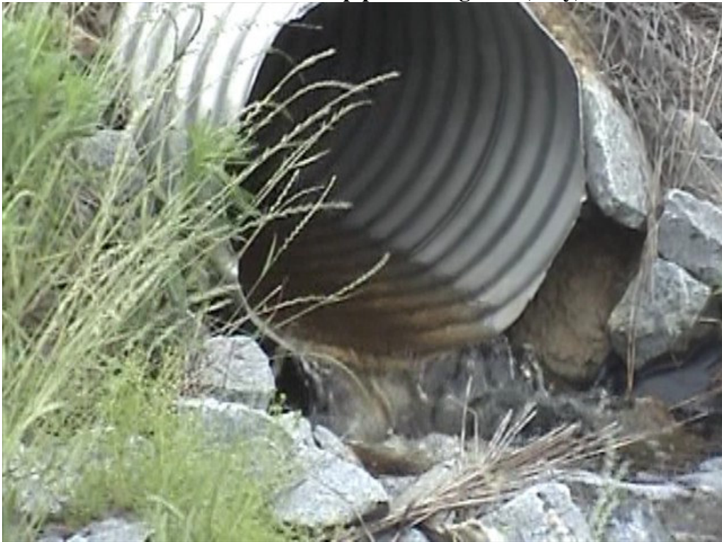
Outflow from outlet pipe showing flow (May)
