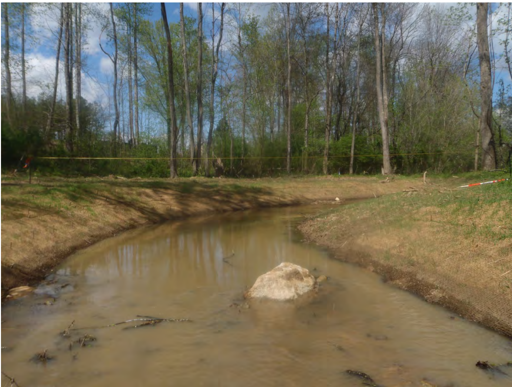
PHOTO AT SECTION 21800
