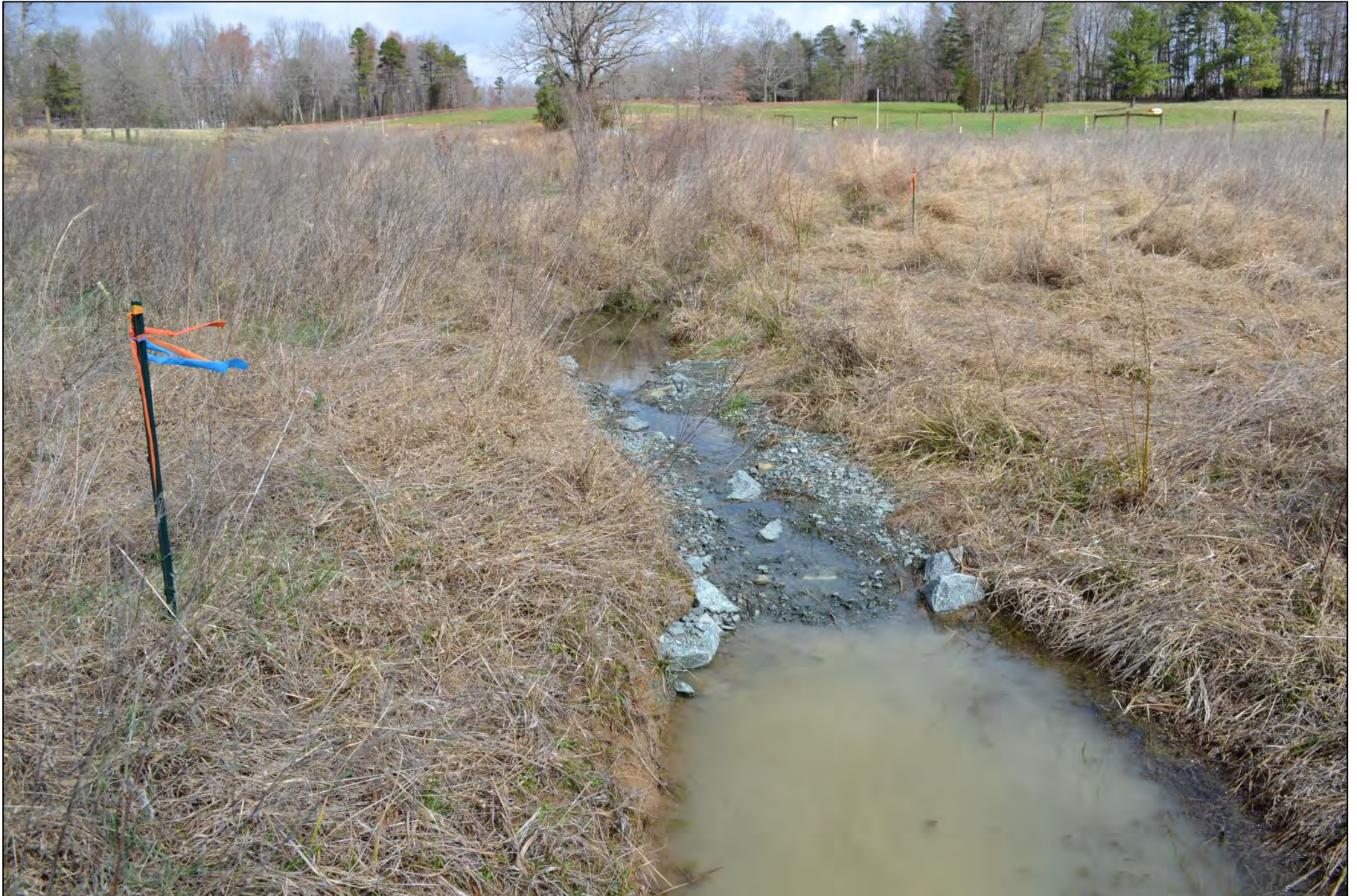
Photo 7: XC-10 – Post 3-1-2017 0.92 inch rain event (Per USGS Gauge at BUFFALO CREEK (SR2819 NR MCLEANSVILLE, NC) ~ 7 miles from Site
