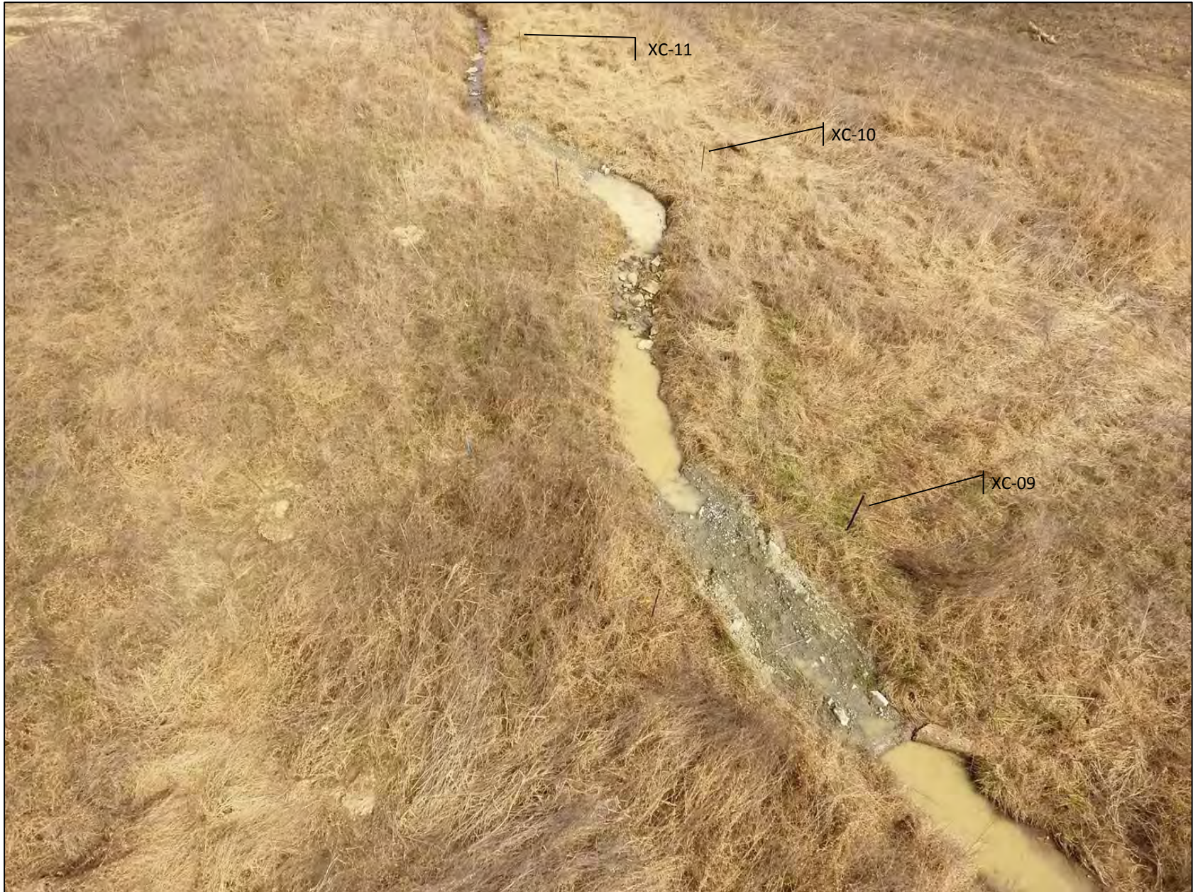
Photo 5: post replacement overview
