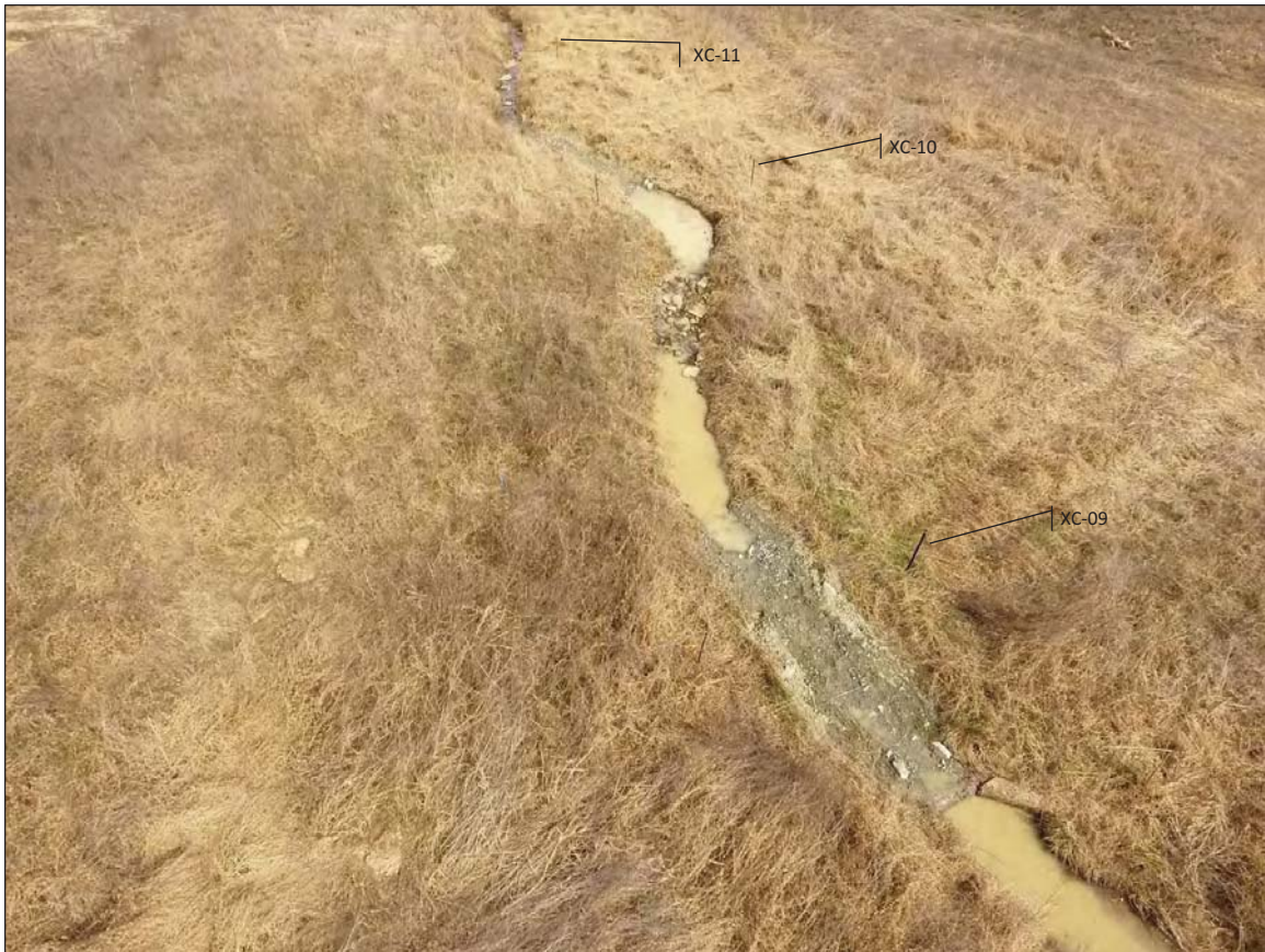
Photo 5: post replacement overview
