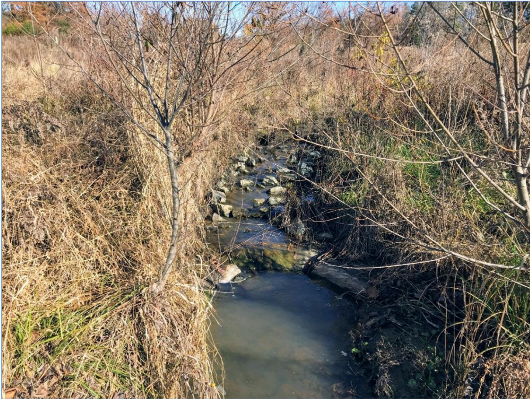
Photo 3: 02-23-2017 Repair near UT-1 XC 9
