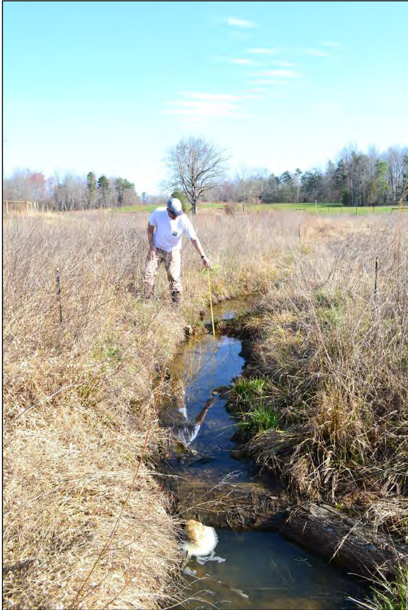
Photo 1: Substrate loss, 6" head-cut at UT 1, XC 9
