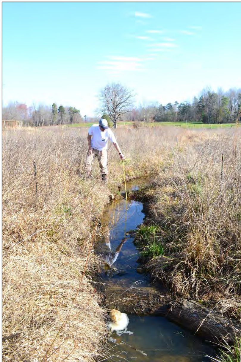
Photo 1: Substrate loss, 6" head-cut at UT 1, XC 9
