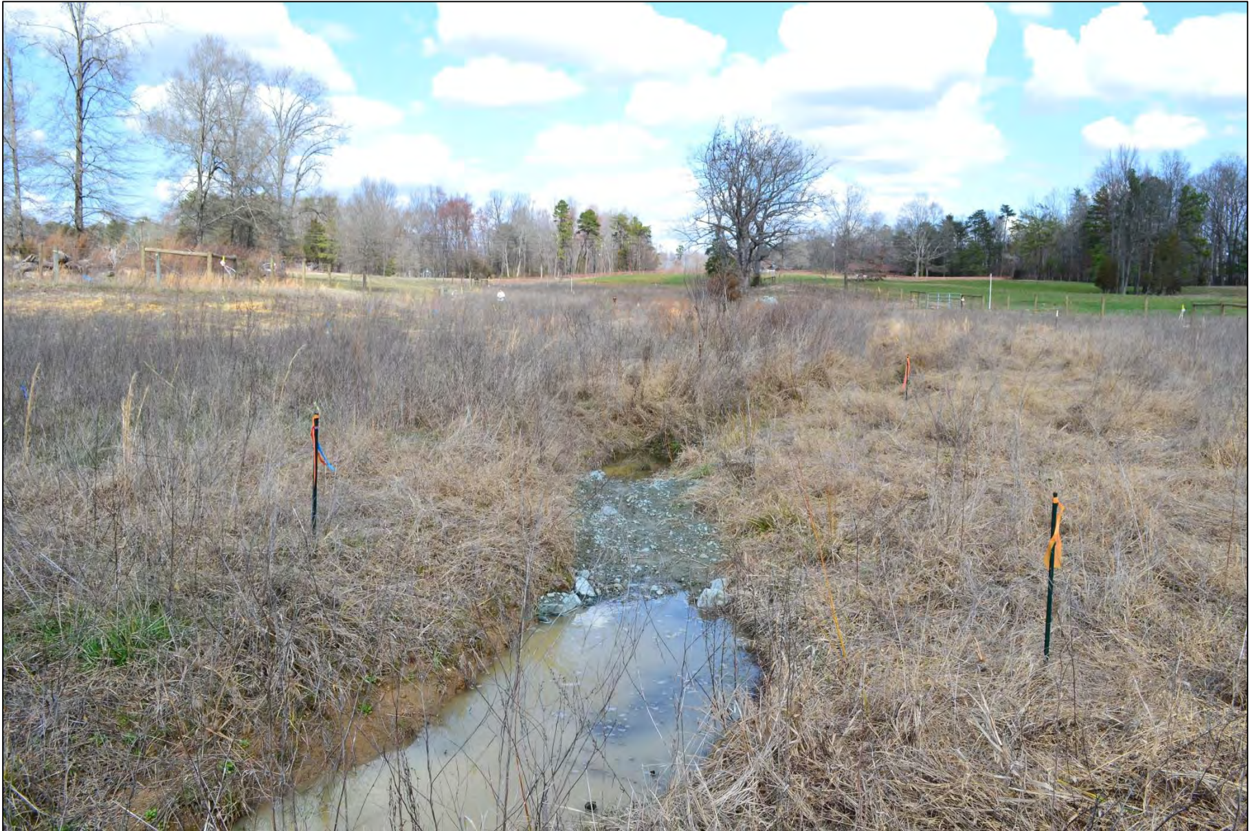
Photo 4: Substrate replaced, upstream riffle of XC 10 (pool)
