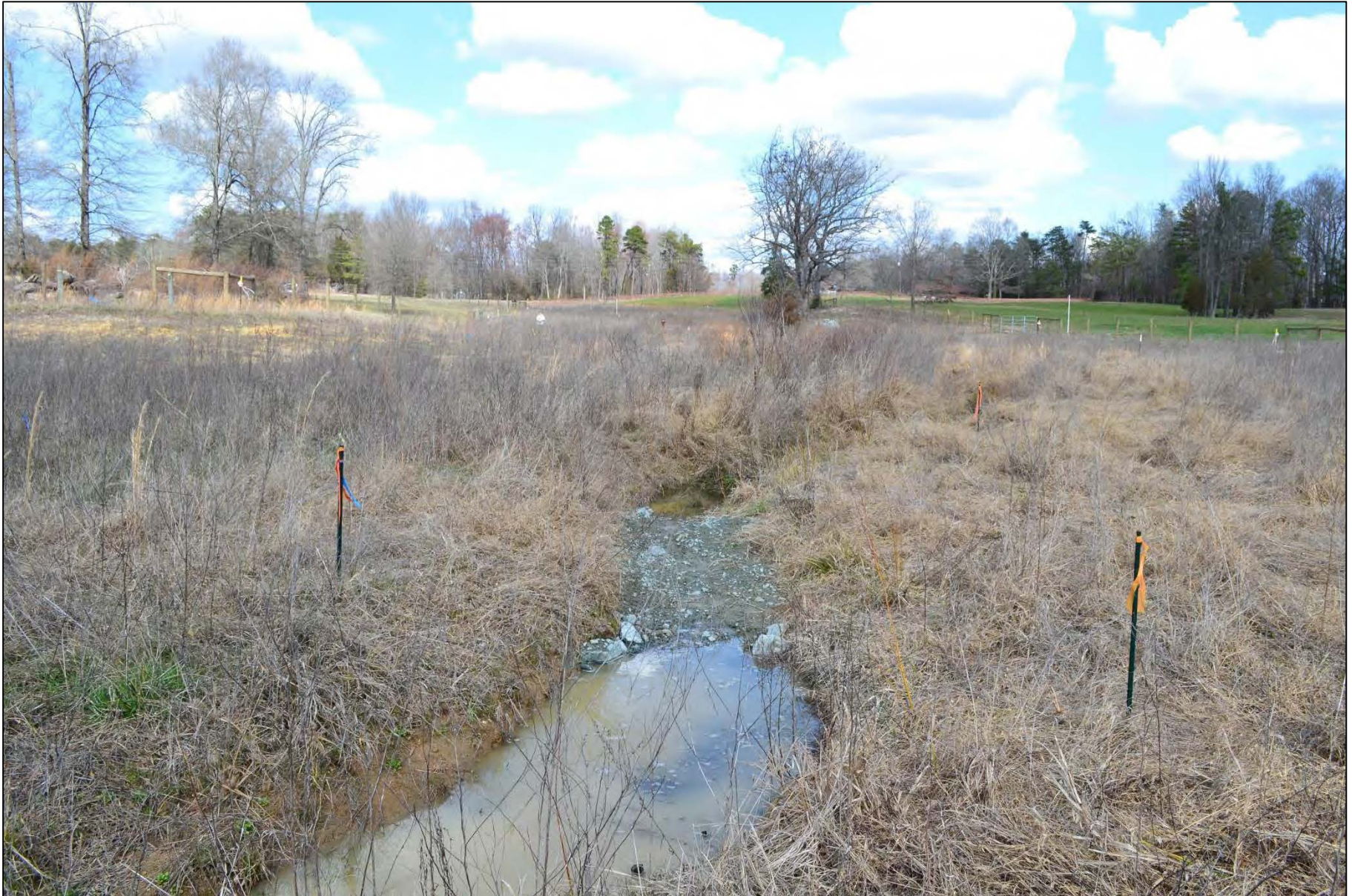
Photo 4: Substrate replaced, upstream riffle of XC 10 (pool)
