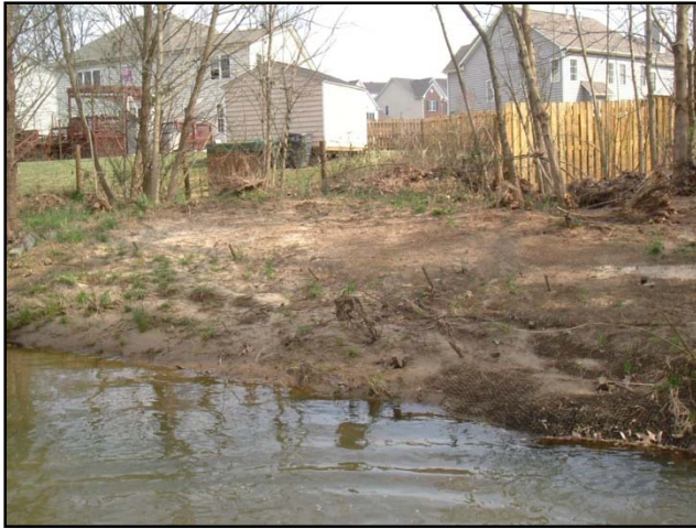
7. Stream Bank Cover Poor 3/22/2007
