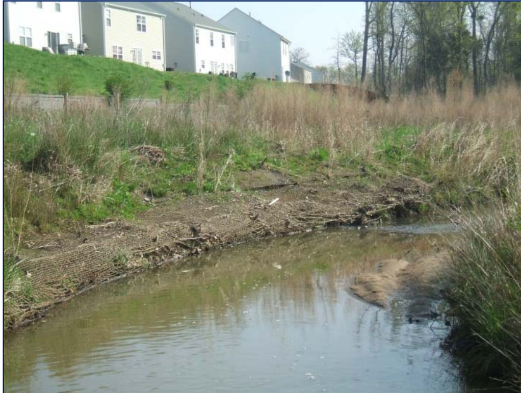
1. Streambank Cover Poor (4/2008)
