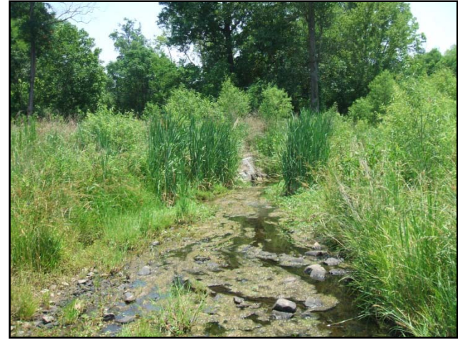
Cross-Section 7-View Downstream Main Channel (4/2008)
