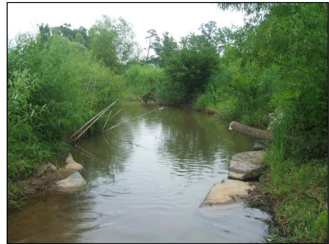
Cross-Section 2-View Downstream Main Channel (6/2009)
