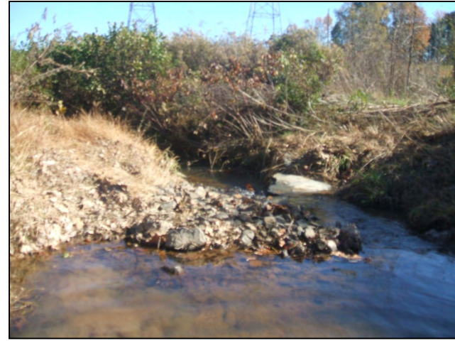
Photo Point 3-View Downstream Main Channel (11/2010)
