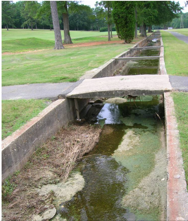
19. Looking downstream. Grass clippings are dumped directly into the stream. Ironically, this has allowed for bankfull formation in the channel, as indicated by the bench on the left side of the stream.
