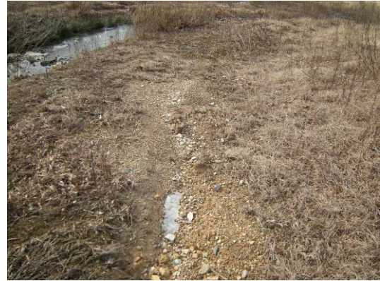
SPA3. Stream overflow channel beginning to form.
