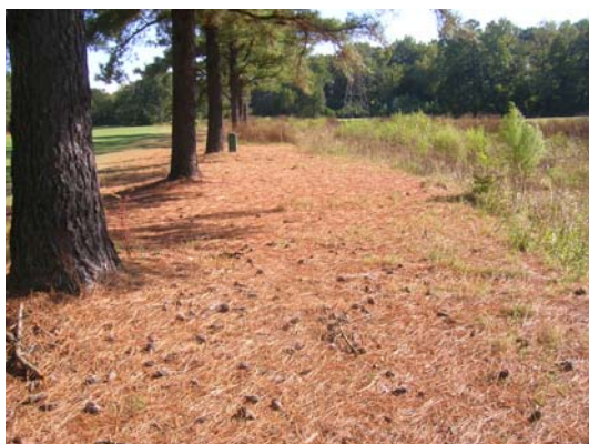
VPA 4. Area of sparse vegetation under mature trees, 39+00 and 42+00.
