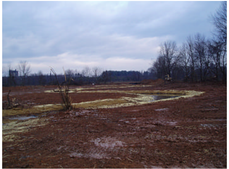
UT3 construction complete_3
