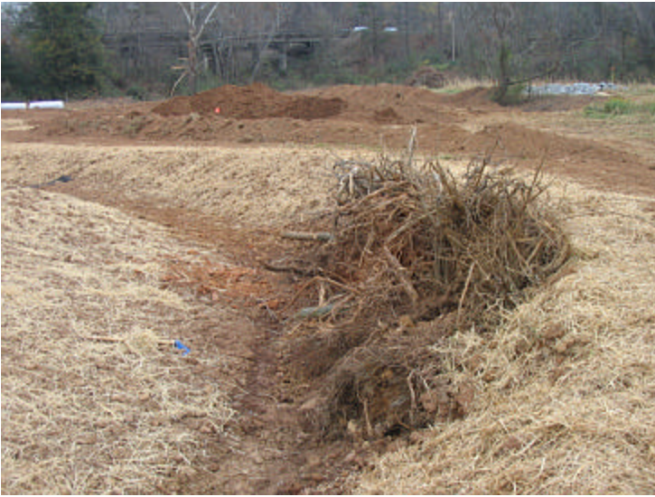
UT2 newly constructed channel_2
