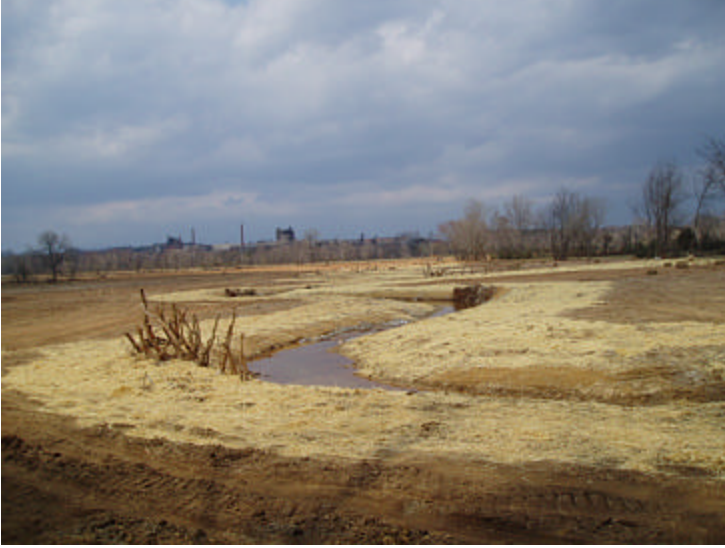
UT3 construction complete_4
