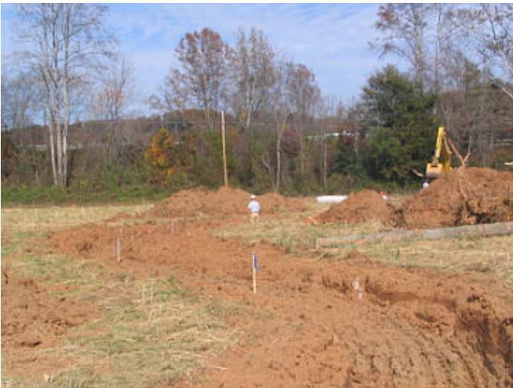
UT1 new channel construction_2
