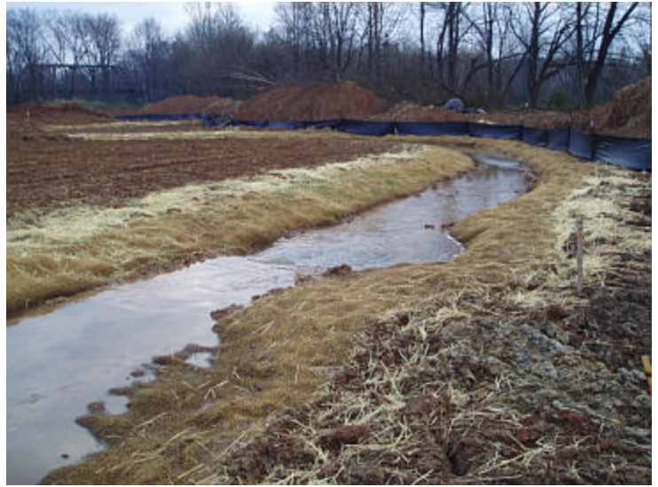
UT3 construction complete_1
