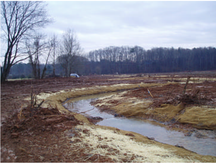
UT3 construction complete_2
