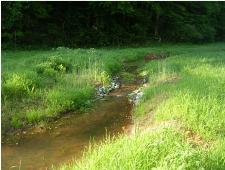
UT1 constructed riffle_3
