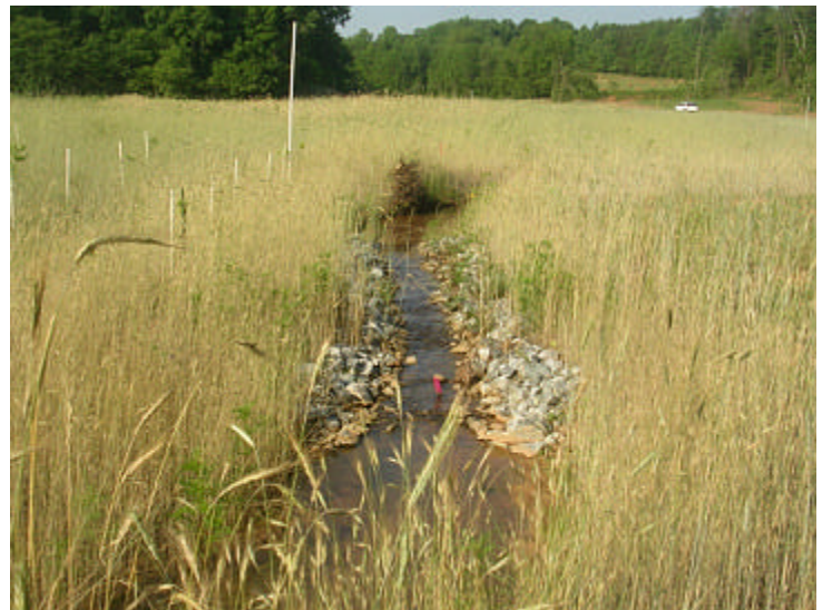
UT2 constructed riffle_1
