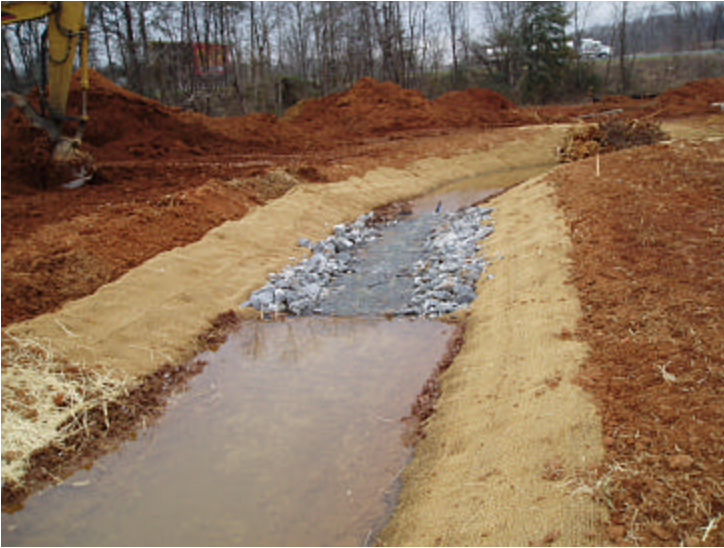
UT1 constructed riffle
