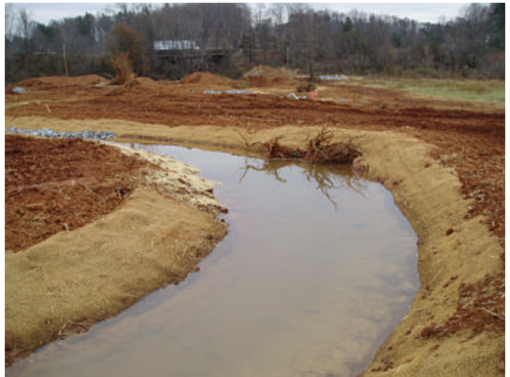
UT1 new channel construction_3
