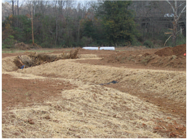
UT2 newly constructed channel_1
