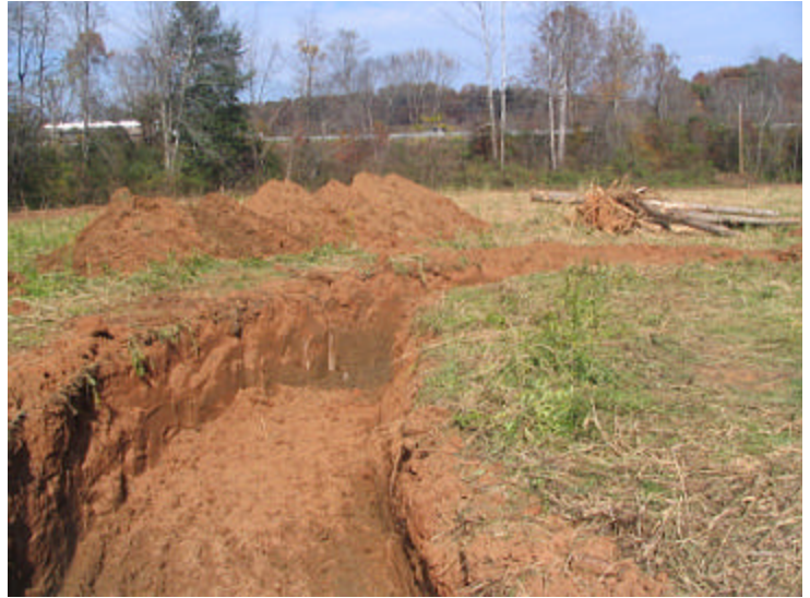
UT1 new channel construction_1
