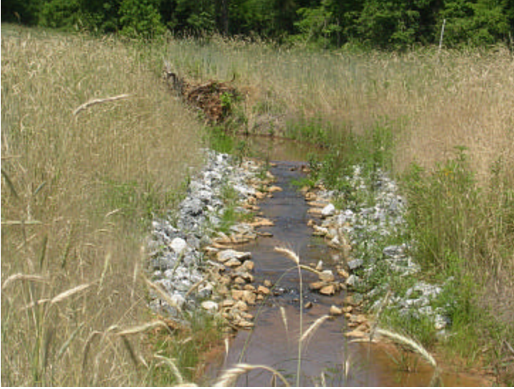
UT1 constructed riffle_1
