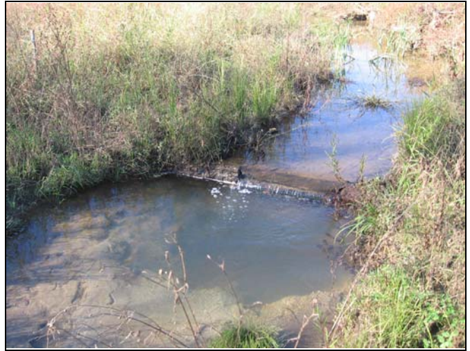
Photo 38 - Log Weir 4 – UT3
