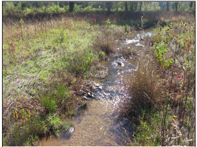
Photo 4 - Constructed Riffle 4 – UT3
