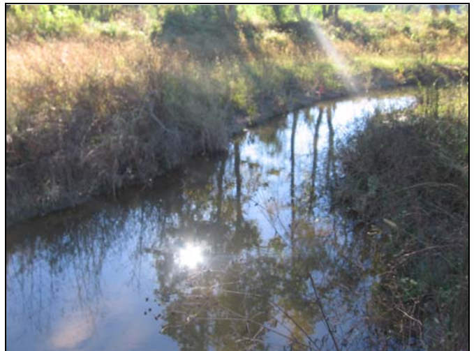
Photo 36 - Log Weir 2 – UT3
