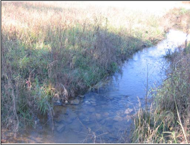
Photo 1 - Constructed Riffle 1 – UT3
