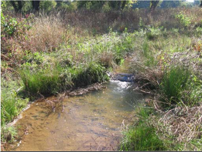
Photo 43 - Log Weir 9 – UT3
