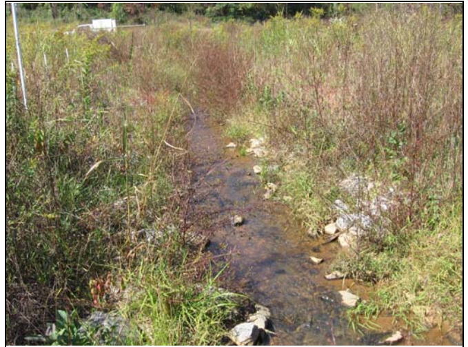
Photo 26 - Constructed Riffle 26 – UT1
