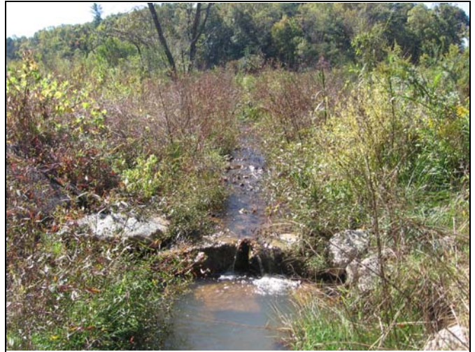
Photo 22 - Constructed Riffle 22 – UT1
