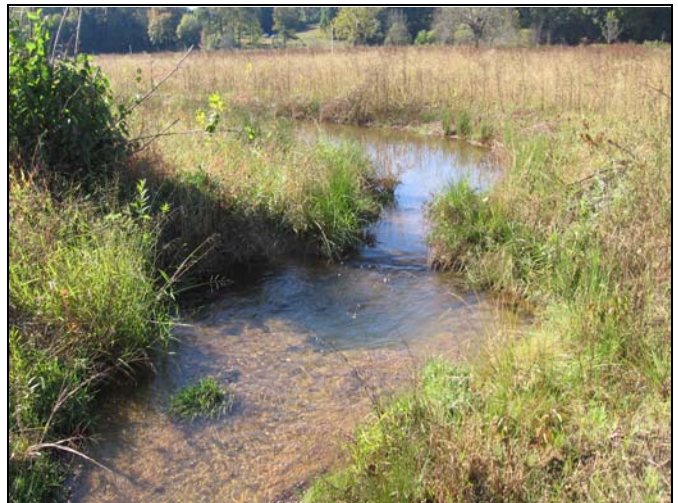
Photo 42 - Log Weir 8 – UT3
