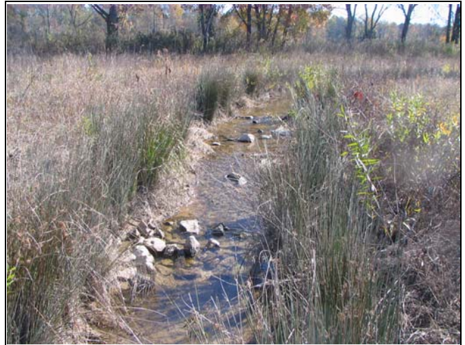
UT3 Constructed Riffle 4
