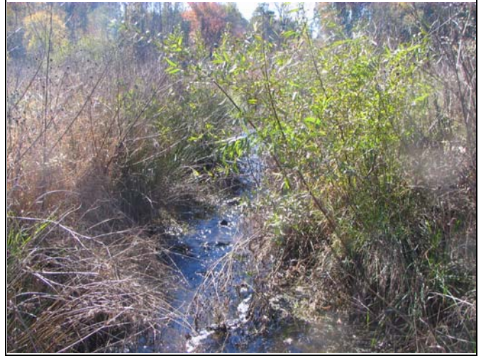
UT3 Constructed Riffle 8
