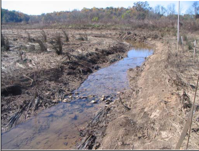
UT3 Constructed Riffle 1
