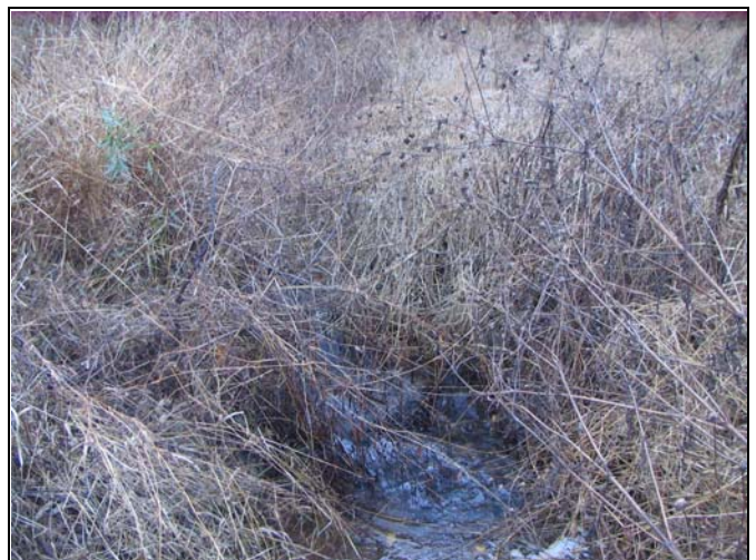
UT1 Constructed Riffle 10
