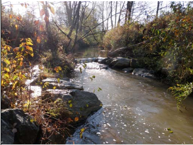
Bailey Fork Cross Vane 1 October (2010) Before repairs
