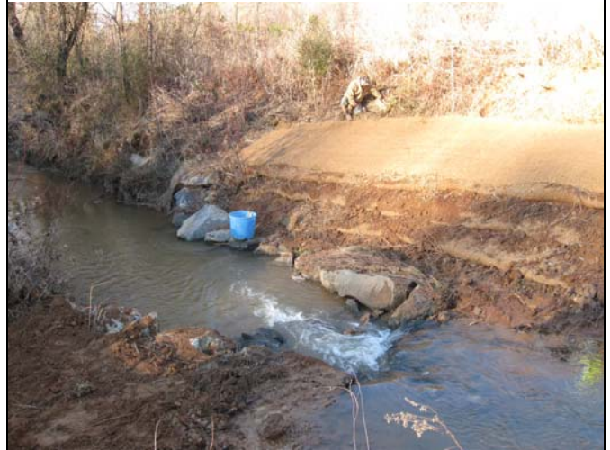
Bailey Fork Cross Vane 1 (December 2010) After repairs
