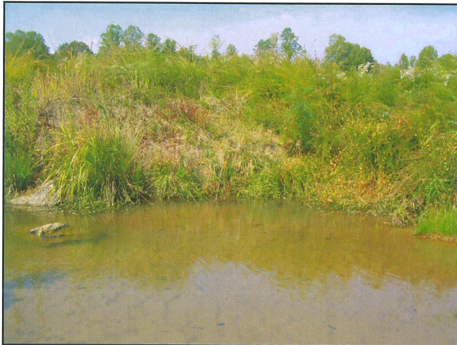
SPA 4 Bank scour in Year 2 along Upper Bailey Fork at station 3+50. Bank is now vegetated. W/D ratio is too high resulting in aggradation. (EMH&T, Inc. 10/22/07)
