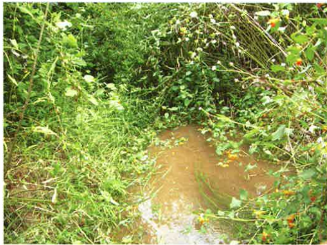
Cross-section photo – looking downstream Channel is obscured by vegetation.
