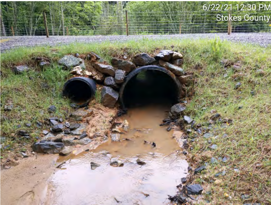
PS-6 – UT1-R2 Culvert Crossing, Upstream (MY-00)
