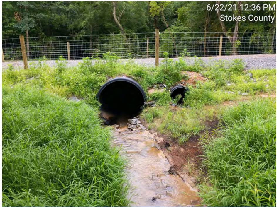
PS-6 – UT1-R2 Culvert Crossing, Downstream (MY-00)
