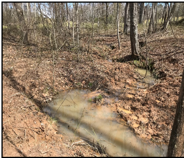
Looking upstream at degraded channel conditions along upper UT1B.
