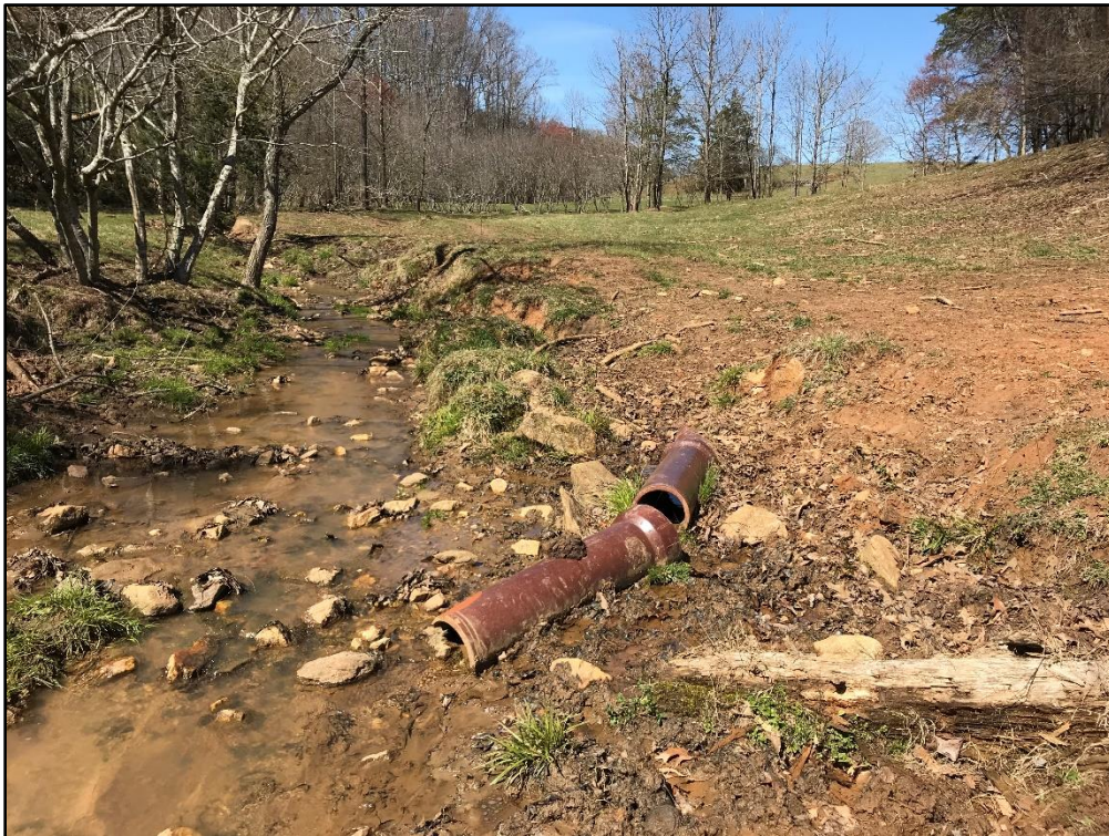
6. Drain tile below W6 wetland.
