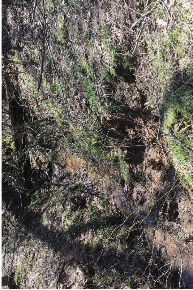
Reach UT1A - Bank erosion due to cattle access
