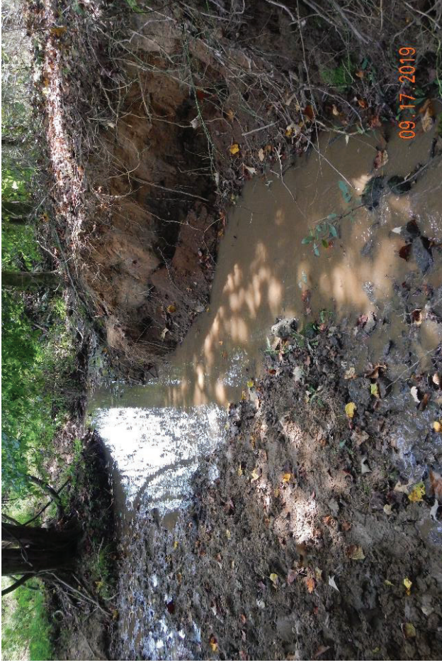
Reach UT1-R2 - Bank erosion and direct cattle access
