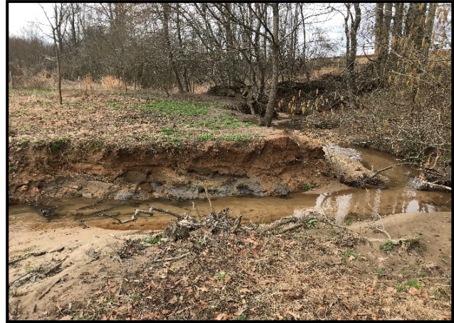
BB-R1 looking downstream. Note the lack of adequate riparian buffer along the left floodplain.
