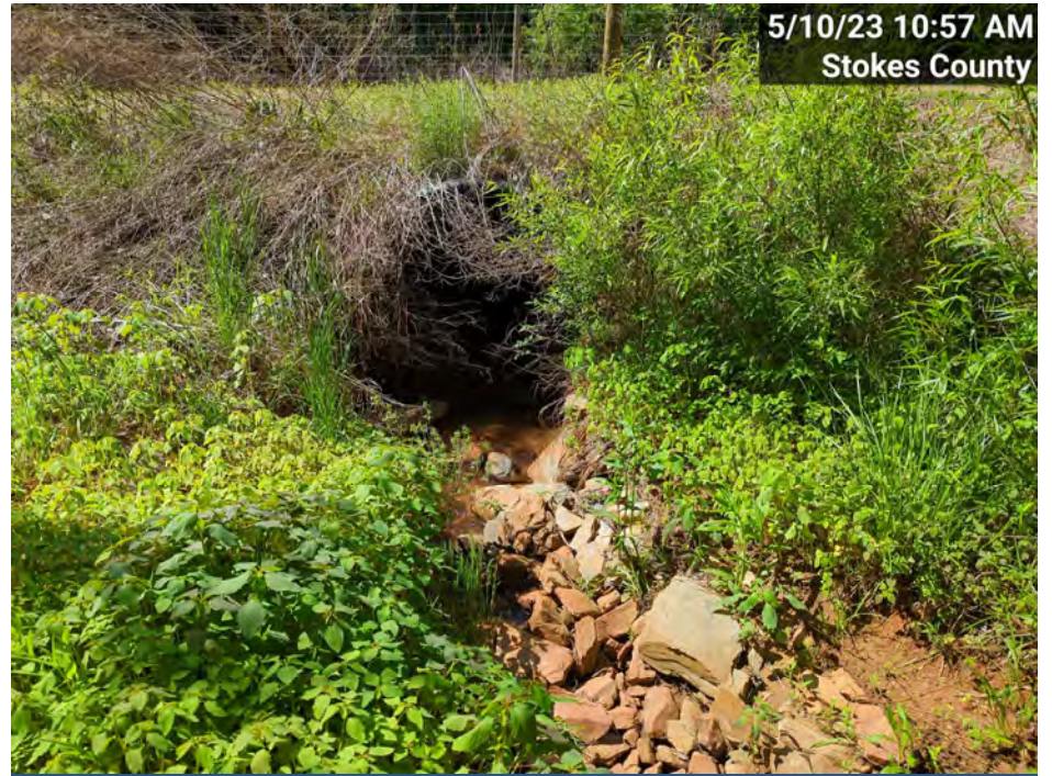
PS-6 – UT1-R2 Culvert Crossing, Downstream (MY-03)
