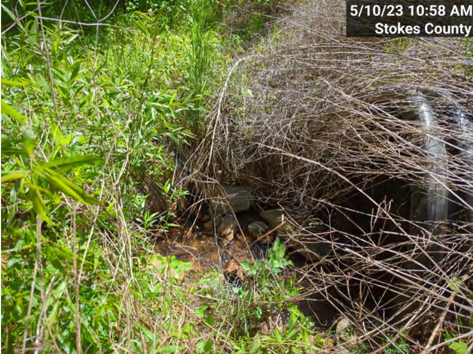
PS-6 – UT1-R2 Culvert Crossing, Downstream Left Bank (MY-03)
