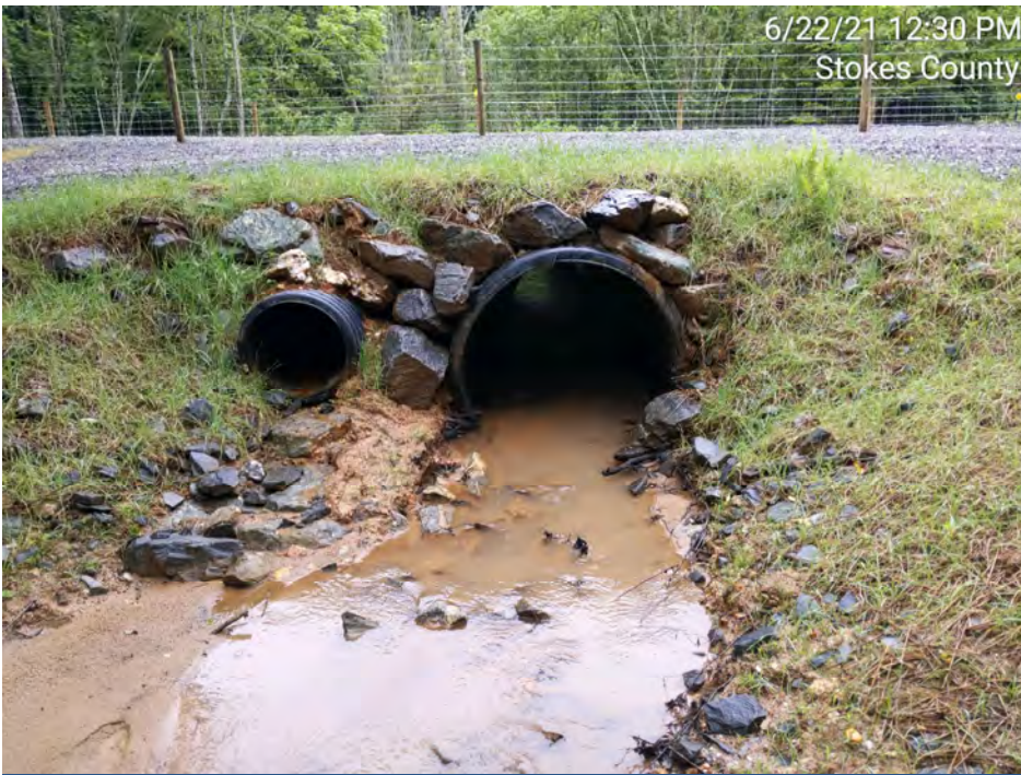
PS-6 – UT1-R2 Culvert Crossing, Upstream (MY-00)
