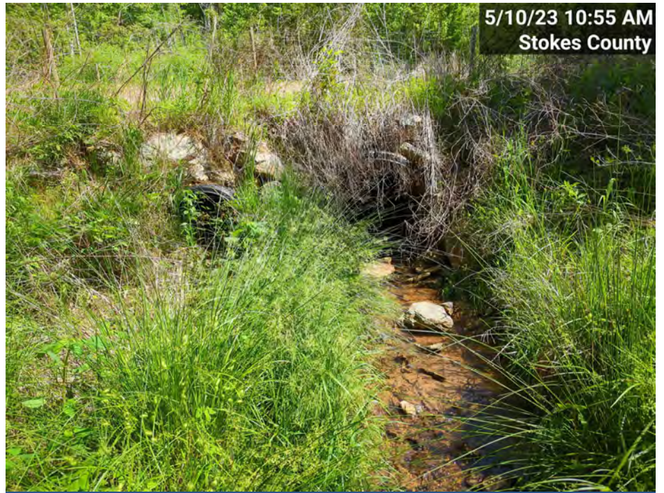
PS-6 – UT1-R2 Culvert Crossing, Upstream (MY-03)
