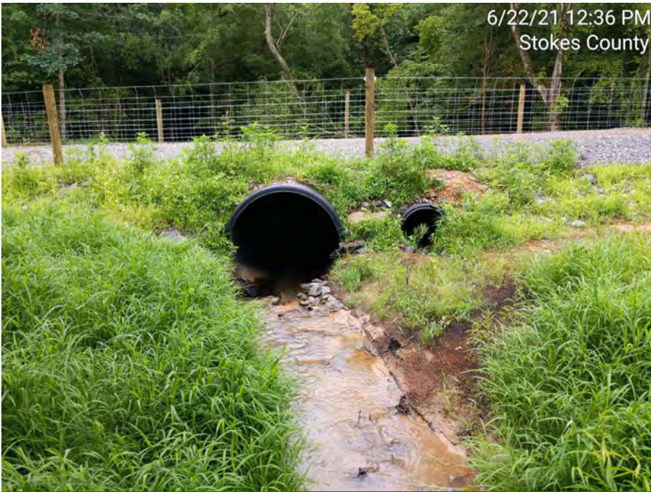
PS-6 – UT1-R2 Culvert Crossing, Downstream (MY-00)
