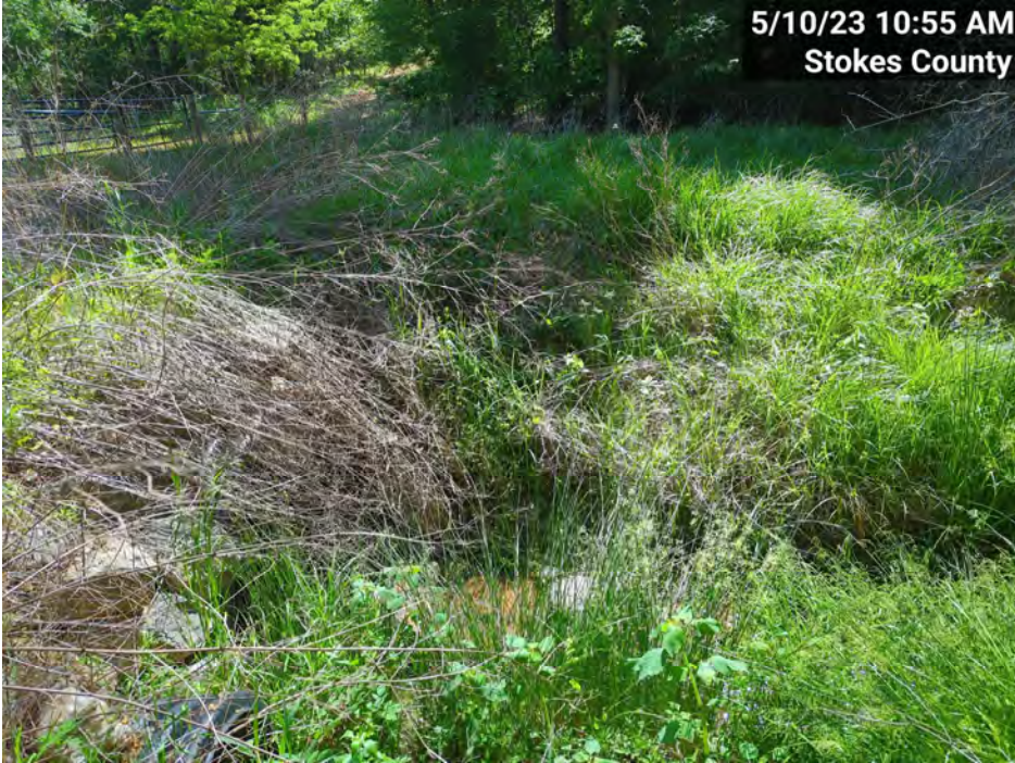
PS-6 – UT1-R2 Culvert Crossing, Upstream Left Bank (MY-03)
