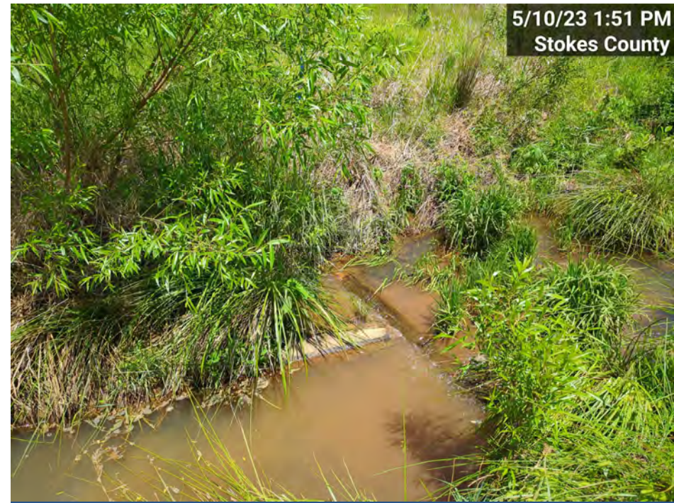
SPA-2 – BB-R3, Erosion around log vane @ STA 70+50 (MY-03)
