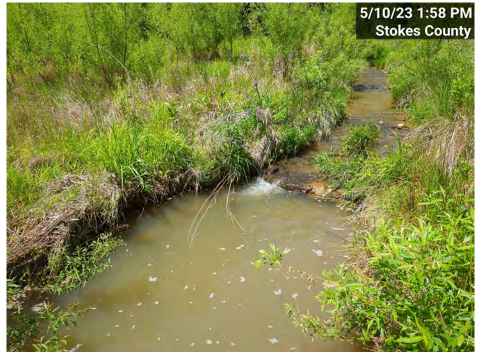
SPA-3 – BB-R3, Rock roller not functioning as intended @ STA 72+00 (MY-03)
