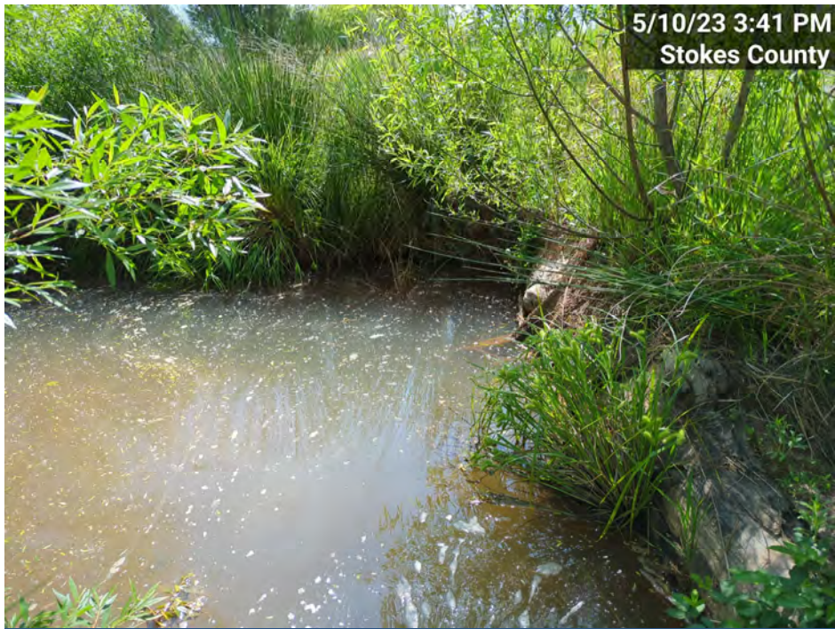
SPA-5 – UT4-R1, Minor erosion downstream of log vane @ STA 51+80 (MY-03)
