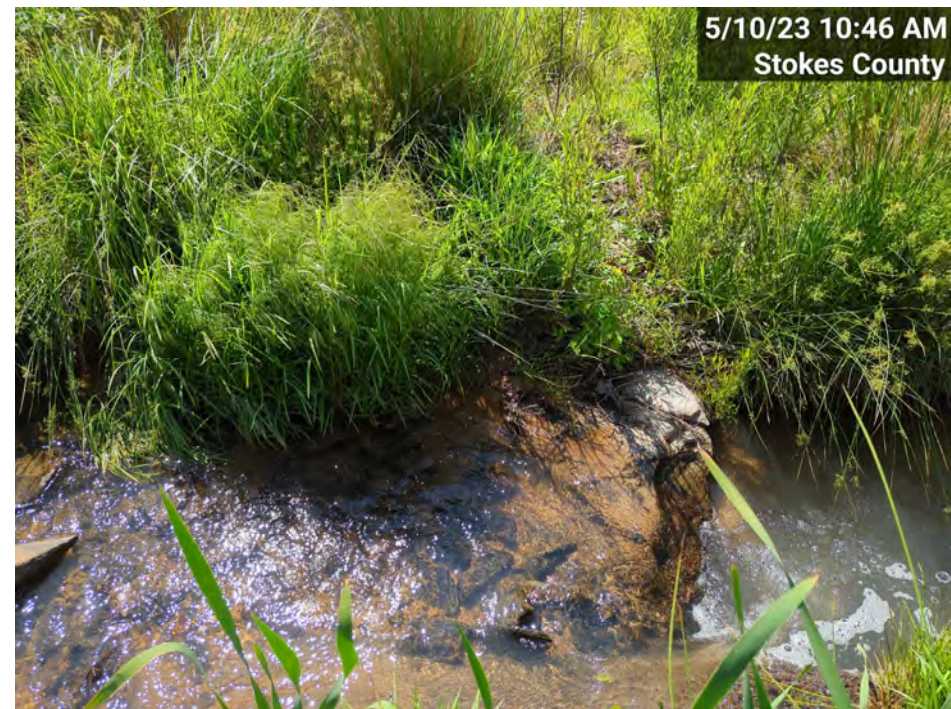
SPA-1 – BB-R1, Piping around rock structure @ STA 44+00 (MY-03)
