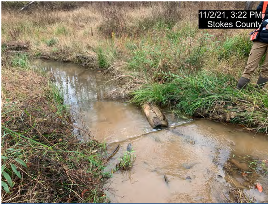
SPA-2 – BB-R3, Erosion around log vane @ STA 70+50 (MY-01)
