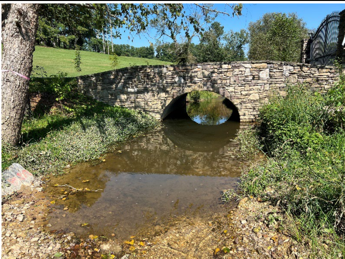
Culvert Crossing – Banner Creek R1, view upstream (09/20/2022)
