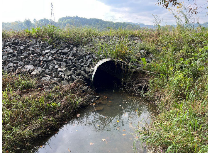
Culvert Crossing – Upper UT1, view downstream (09/20/2022)
