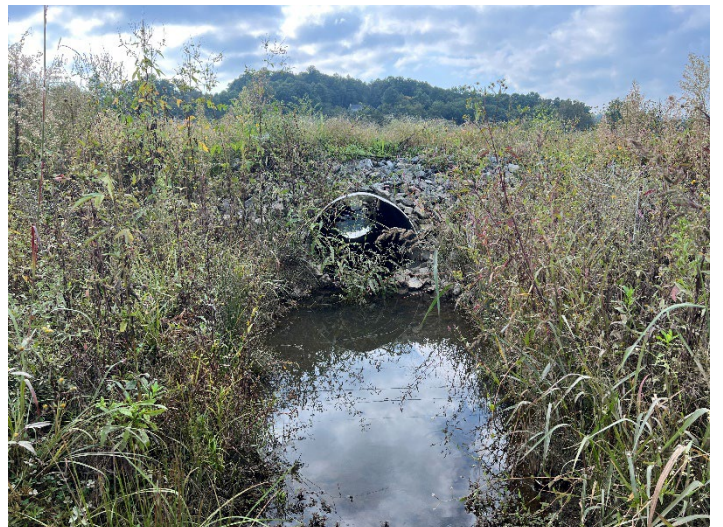
Culvert Crossing – Lower UT1, view downstream (09/20/2022)
