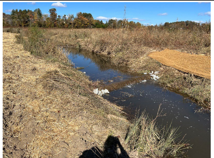
Post-repair: BC R4b, STA 35+85, structure & bank repair (10/19/2022)
