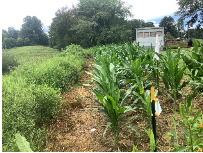
Easement Encroachment - Unresolved: Banner Creek Reach 2 STA 15+00, Left floodplain boundary, Garden row crop overreach (07/14/2022)
