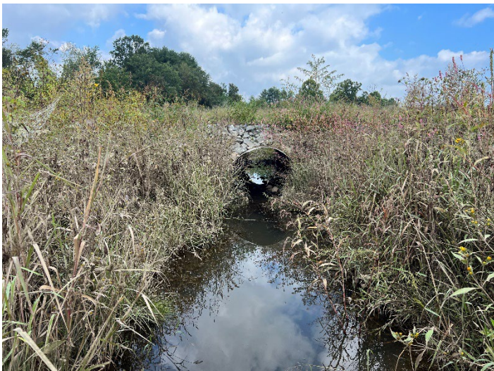
Culvert Crossing – Lower UT1, view upstream (09/20/2022)
