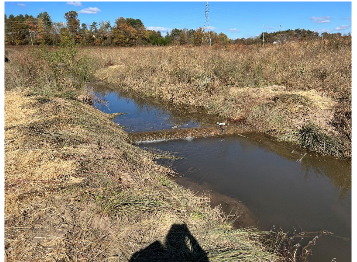
Post-repair: BC R4b, STA 35+25, structure & bank repair (10/19/2022)
