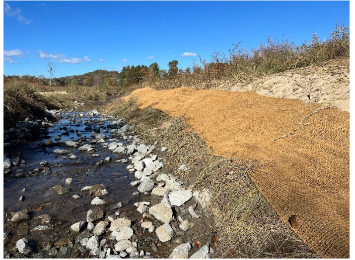
Post-repair: BC R4b, STA 37+00, riffle & bank repair (10/19/2022)
