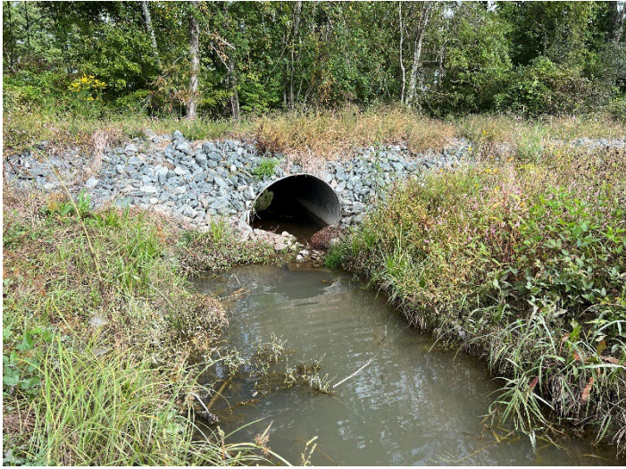
Culvert Crossing – Upper UT1, view upstream (09/20/2022)
