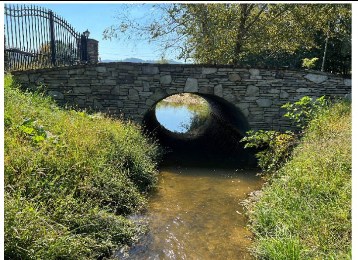
Culvert Crossing – Banner Creek R1, view downstream (09/20/2022)
