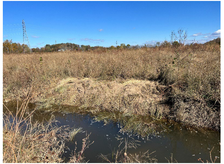
Post-repair: BC R4b, STA 34+55, left bank repair (10/19/2022)
