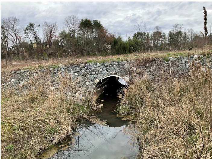
Culvert Crossing – Lower UT1, view upstream (03/08/2023)
