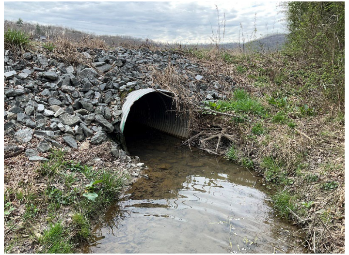
Culvert Crossing – Upper UT1, view downstream (03/08/2023)
