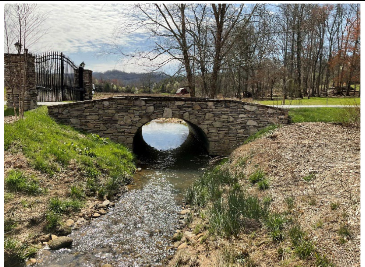
Culvert Crossing – Banner Creek R1, view downstream (03/08/2023)
