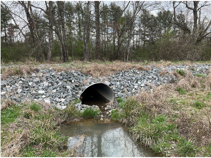
Culvert Crossing – Upper UT1, view upstream (03/08/2023)
