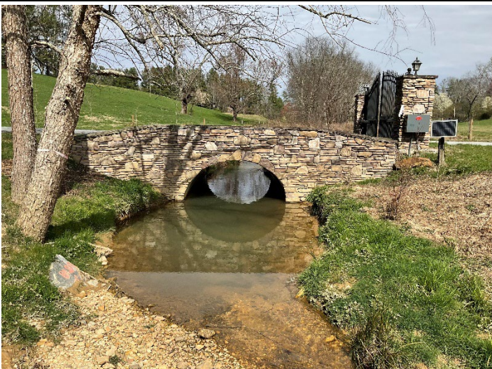
Culvert Crossing – Banner Creek R1, view upstream (03/08/2023)
