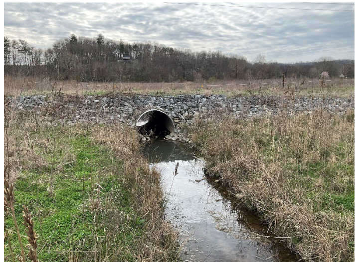
Culvert Crossing – Lower UT1, view downstream (03/08/2023)
