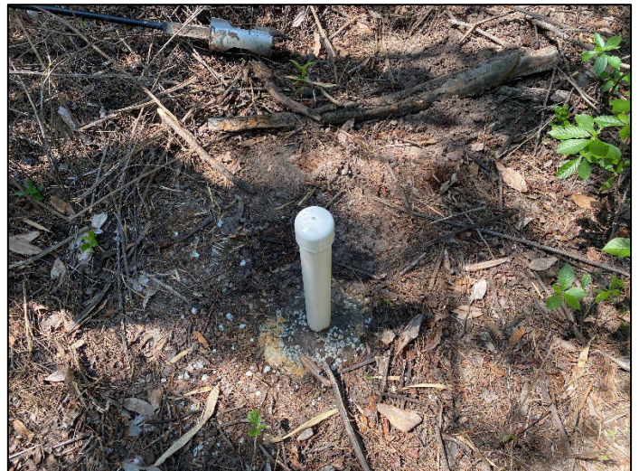
Groundwater Well 14 Reinstall (05/19/22)
