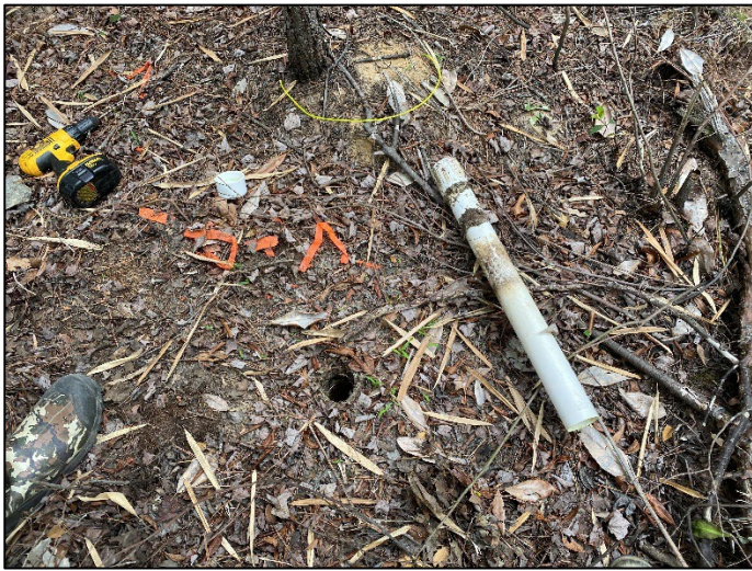
Broken Groundwater Well 14 (05/12/22)
