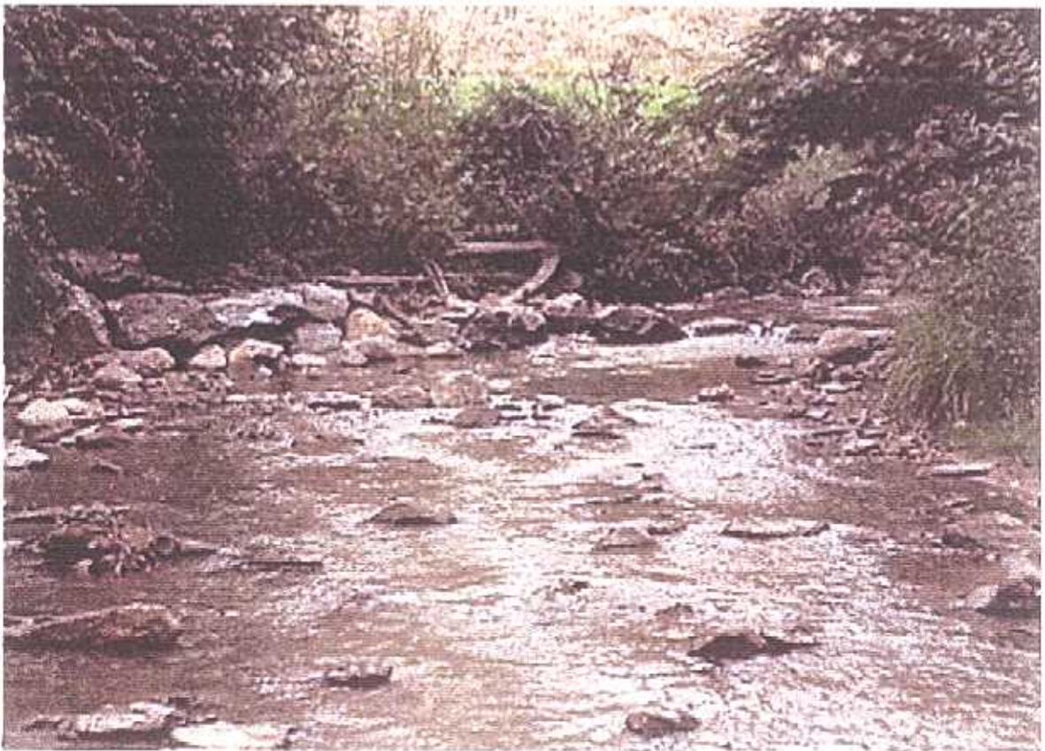
Site of second vane, taken from the third vane upstream. Top photo shows the area before construction and bottom photo shows the same area after construction, with scour hole developed.
