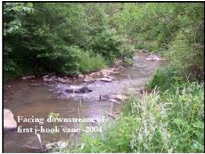
Photo sta. 2, facing downstream, May 2004.
