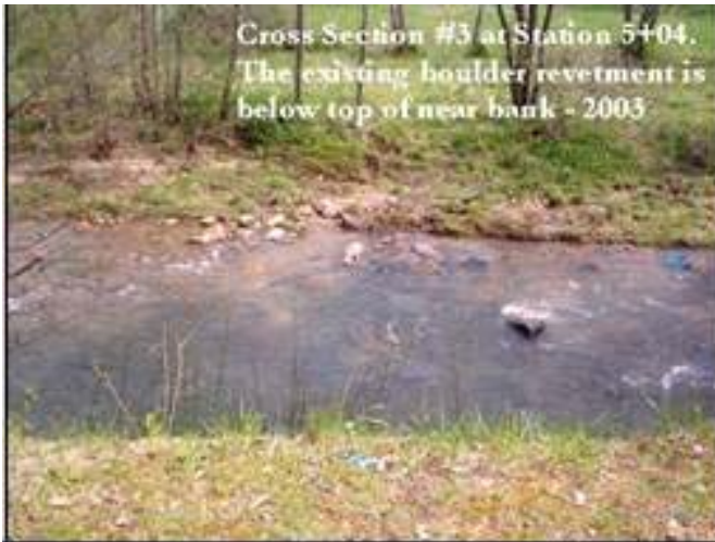
Cross-section 3, right bank to left bank, March 2003.
