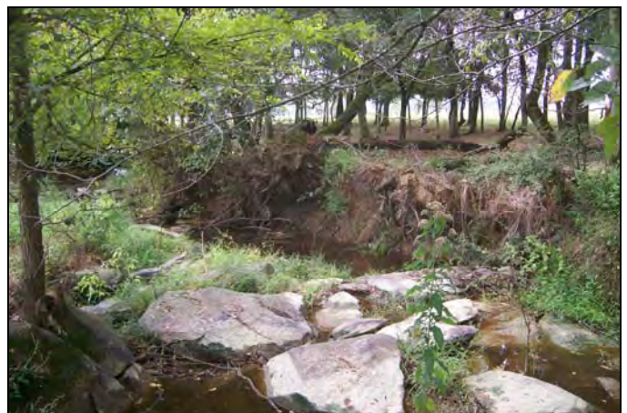
Photo 6-View of right bank erosion on Bear Creek Reach B, facing downstream.
