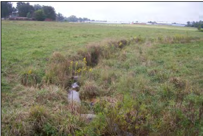
Photo 9-View of UT to Bear Creek, facing upstream from Siler City Glendon Road.
