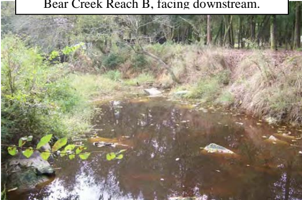
Photo 5- View of erosion along right bank of Bear Creek Reach B, facing downstream.
