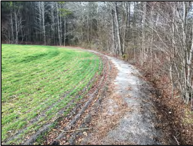
North end of project, showing existing swale where ditch off-site will be reconnected.
