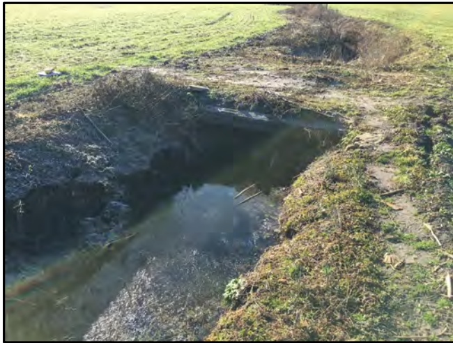
View of existing crossing, looking upstream.
