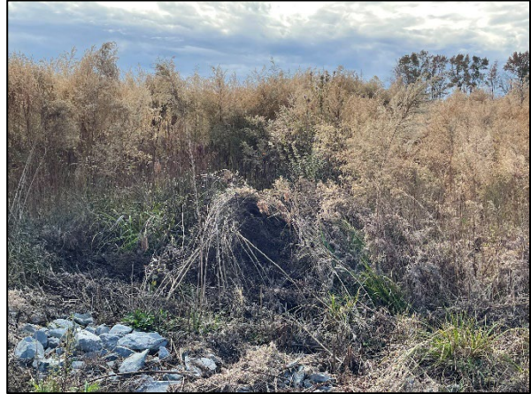
Photo Point 2 – Sta. 10+00 Facing Downstream (11/23/2022)
