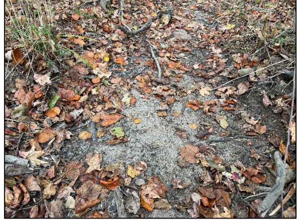
Evidence of channel formation: sediment deposition in channel (10/26/2022)
