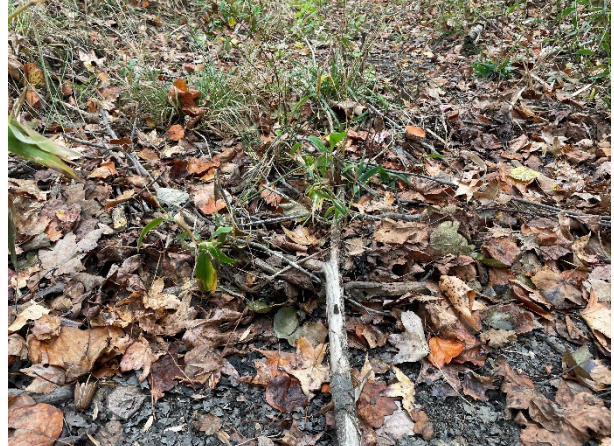
Evidence of channel formation: wracking and debris (10/26/2022)
